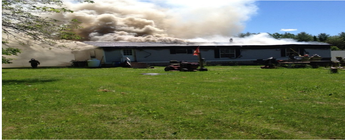
Clinton Mobile Home Fire
