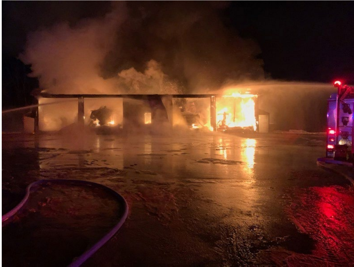
Fort Fairfield Maine DOT Building: January 2, 2020
