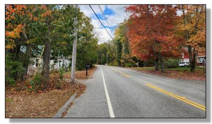
curbed with closed drainage near the intersection and uncurbed with open drainage away from the intersection. There are overhead utilities and utility poles along the corridor. The roadway has a relatively flat profile with a horizontal curve near the study limits. There are residential properties along this section of the roadway. There are intersections with Kathy Lane and Tammy Lane along this section of Skillin Road.
