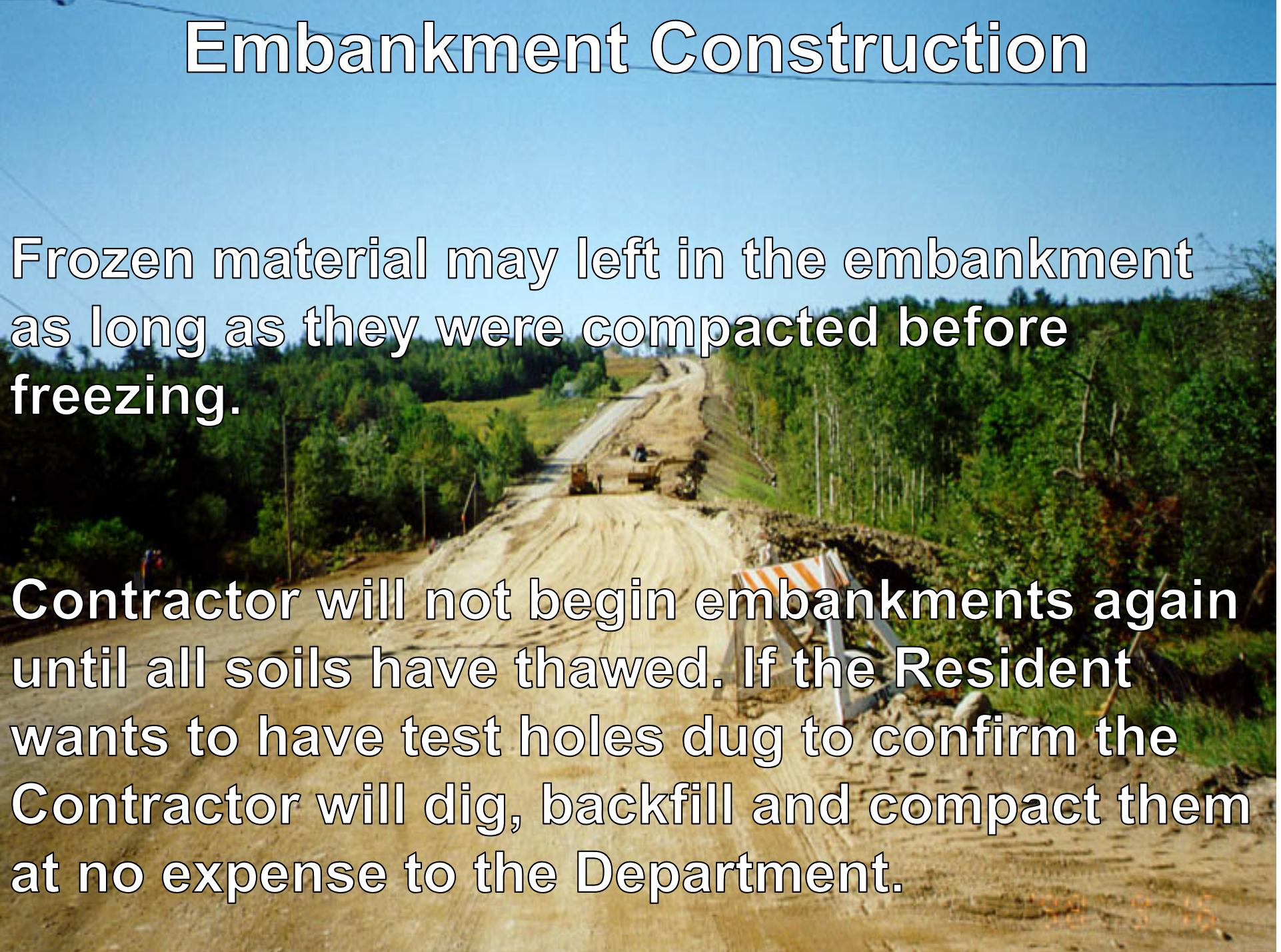
Frozen material may left in the embankment as long as they were compacted before freezing.
