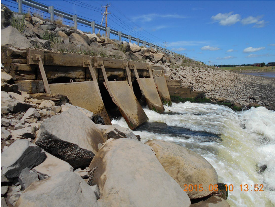
Photo 2. Existing tide gates during a low tide in the Machias River Estuary
