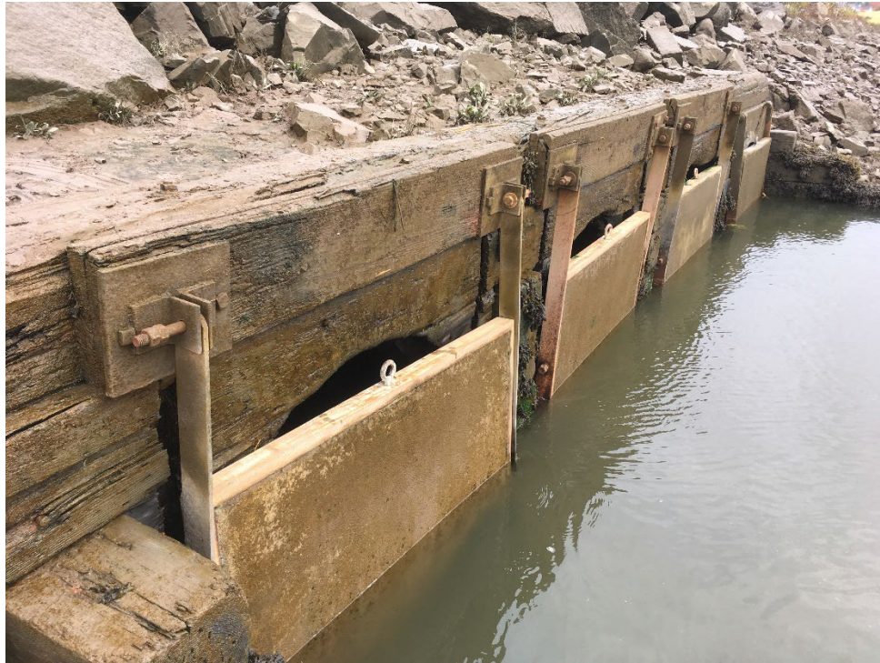
Photo 16. Looking east at tide gates on an incoming tide.
