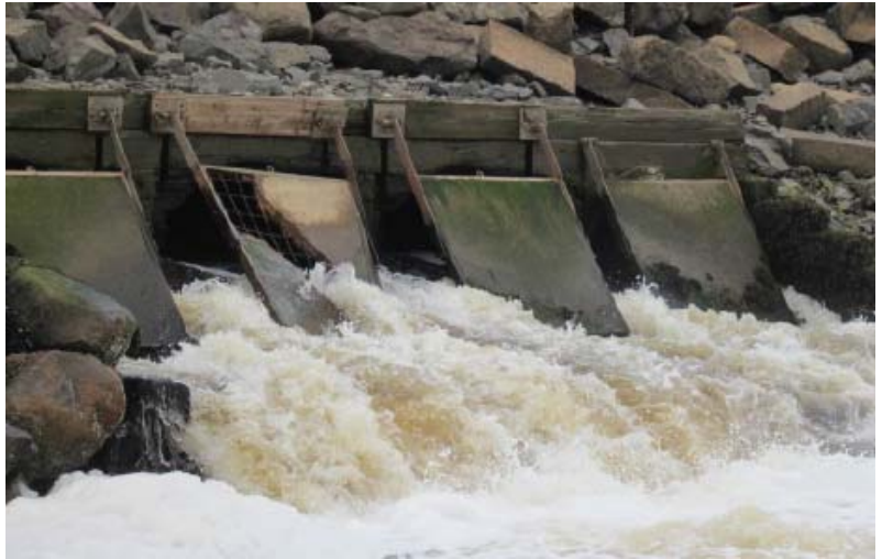
Photo 2. Dyke Bridge culverts with flap gates.
