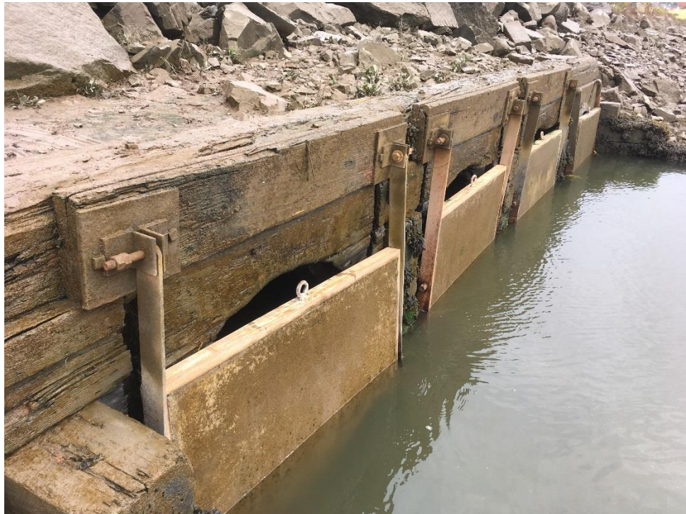
Photo 1. Looking east at tide gates on an incoming tide.
