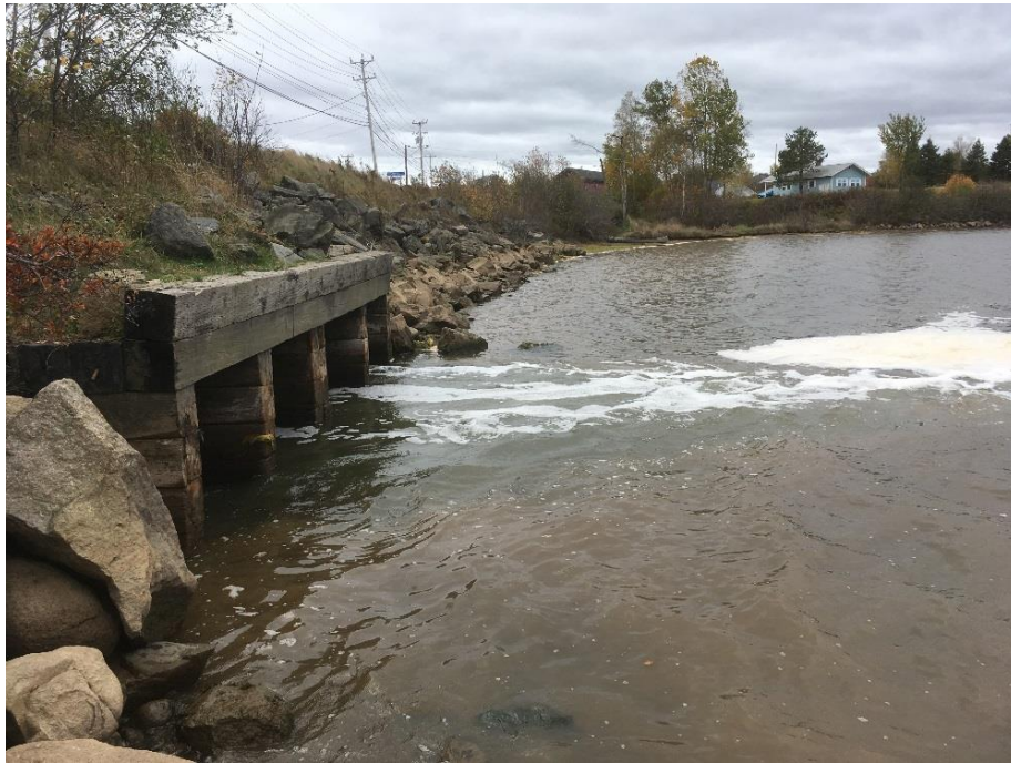
Photo 4. Middle River box culvert and riprap shoreline during rising tide
