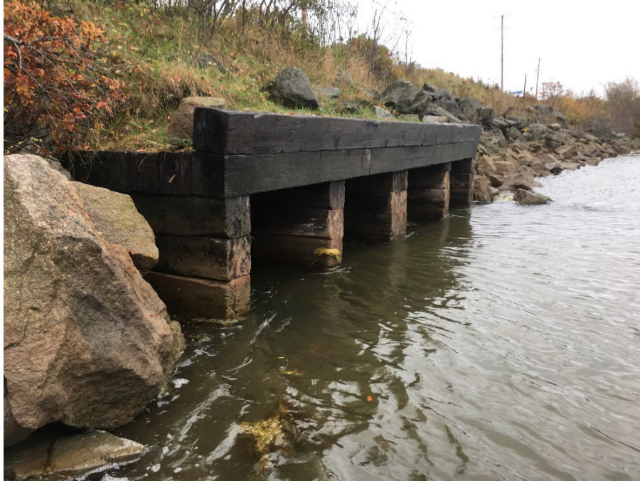
Photo 3. Middle River box culvert and riprap shoreline during falling tide (Stantec 2017)
