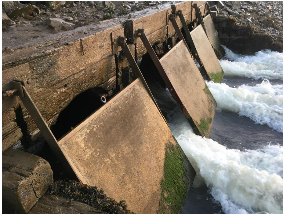
Photo 15. Looking east at tide gates on an outgoing tide.
