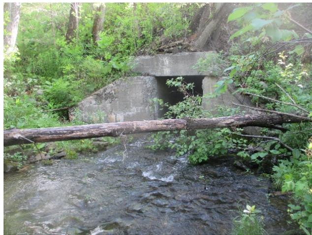
In addition to wildlife crossing concerns, physical elements of the culvert are also failing including the existing inslopes, wingwalls and gabion walls. Debris is also accumulating at the inlet end of the culvert. During one major weather event in 1983, the entire roadway flooded likely due to the Project being at the bottom of two significant downslopes.
