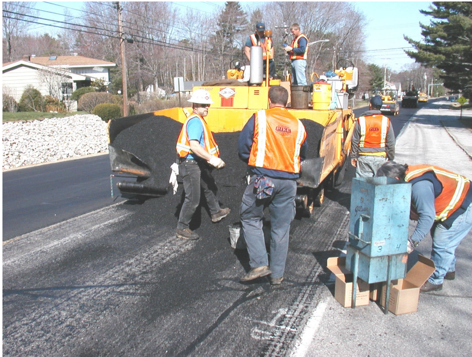
Paving Inspector loads the Quartermaster splitter.
