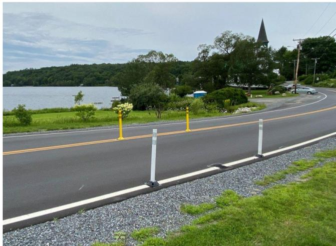
*Short segment of Tuff Curb to be used with/instead of a flex-post*
