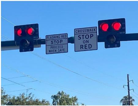
**Figure 11 – Pedestrian Hybrid Beacon (PHB)**
