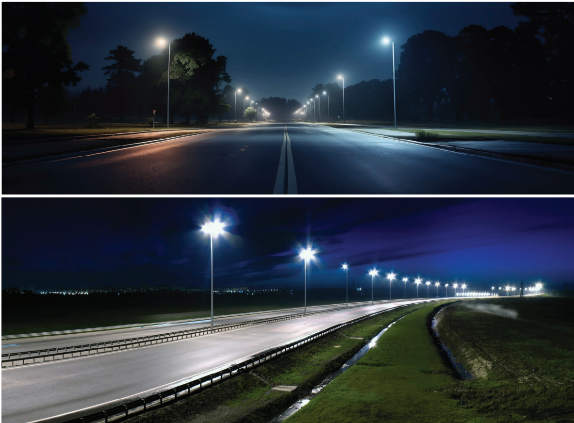
Figure 2-17. Photos. Examples of roadway lighting uniformity. (Top) Poor roadway uniformity (>6:1). (Bottom) Good roadway uniformity <4:1).
