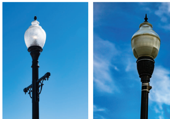
Figure 2-23. Photos. (Left) Roadway luminaire with new clean glass refractor. (Right) Roadway luminaire dirt depreciation.
