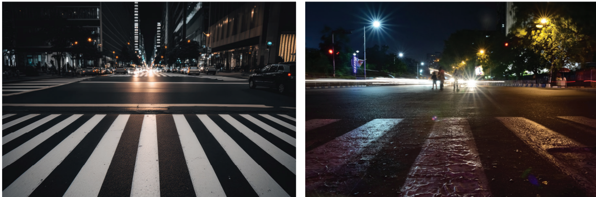
Figure 2-20. Photos. (Left) A newly painted crosswalk with high luminance ratio for striping. (Right) An older crosswalk with low luminance ratio for striping.
