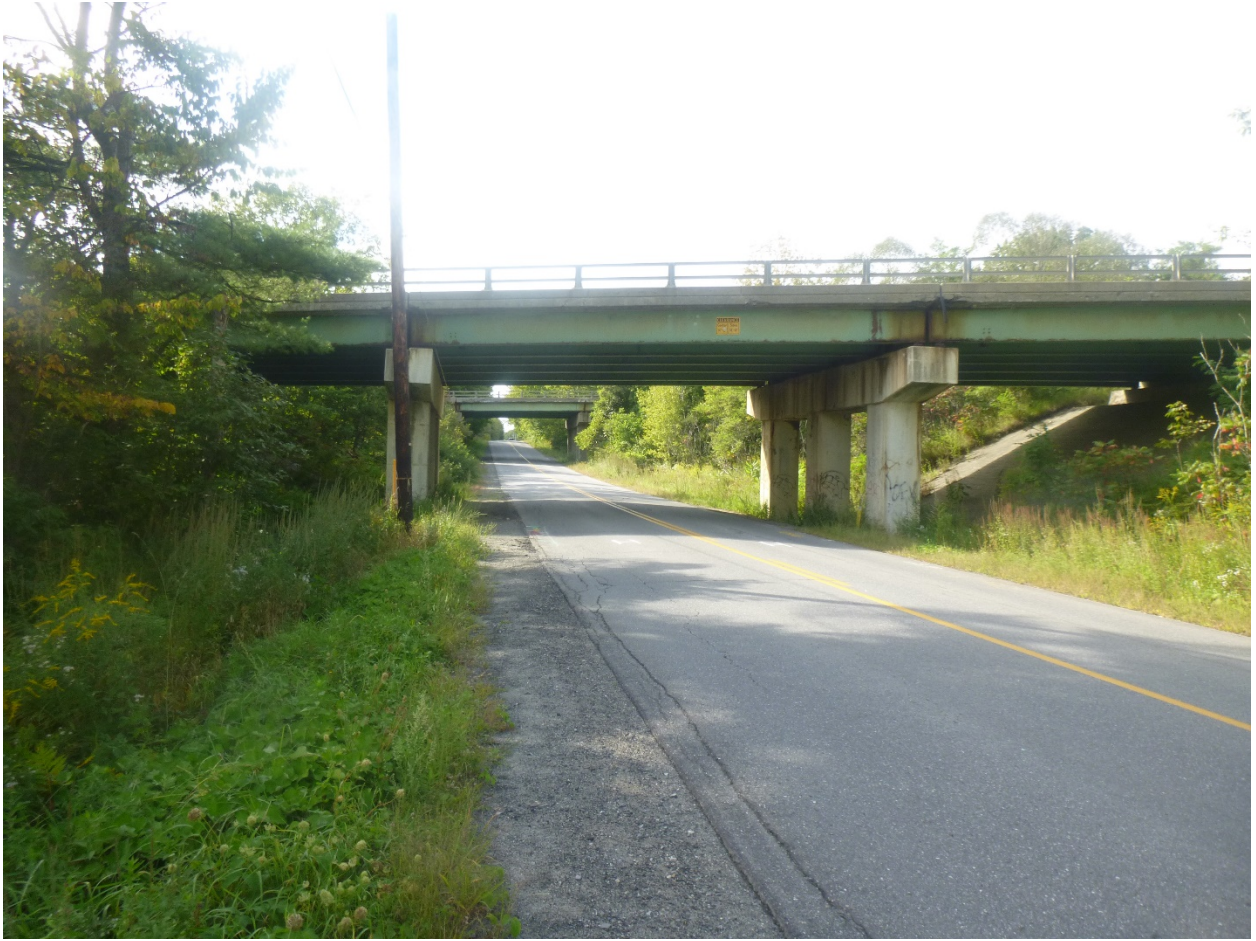
I-95 / Webb Road Bridges in Waterville
