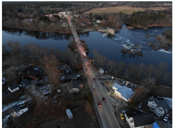
Aerial View of Stillwater Bridges
