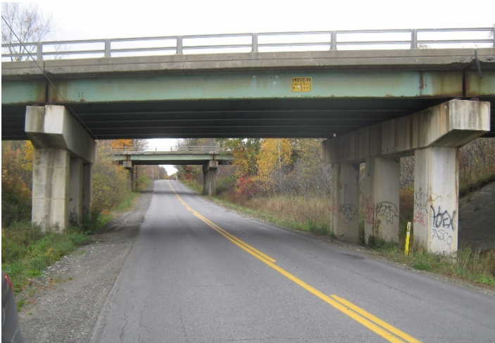
I-95 / Webb Road Bridges from Webb Road
