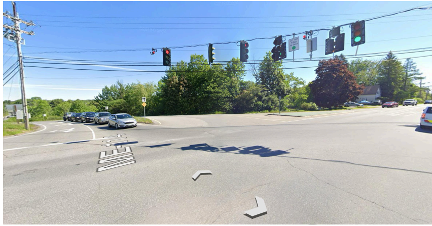
Intersection of South Street and County Road in South Gorham. Here, a slip lane was added to speed vehicles turning north from the overlap. Again, there is ample space for a roundabout, and the traffic signals in the area are outdated. Image from Google Street View, July 2023, day and time unknown.
