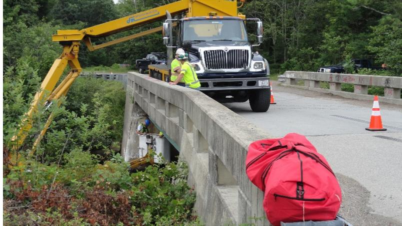
Figure 3: MaineDOT UBIT utilized to install sensors
