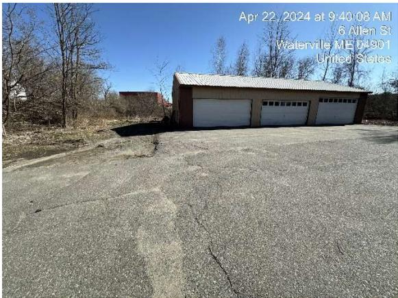
*KVCAP Existing Conditions including a deteriorating facility roof and parking lot area in need of weatherproofing.*
