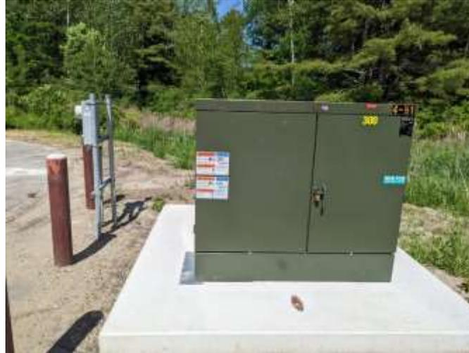
**Figure 9 Dedicated Transformer for BEB Chargers at 13 Pomerleau St.**
