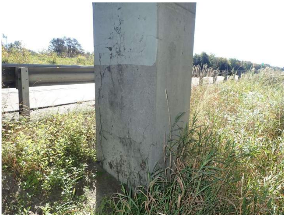
PHOTO 56 Condition Description Pier 1 - cracking, map cracking on column at ground level
