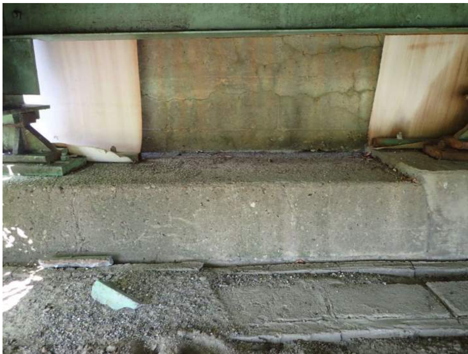
PHOTO 42 Condition Description Abutment 1 - bay 3, girders 4 & 3, moderate cracking on backwall
