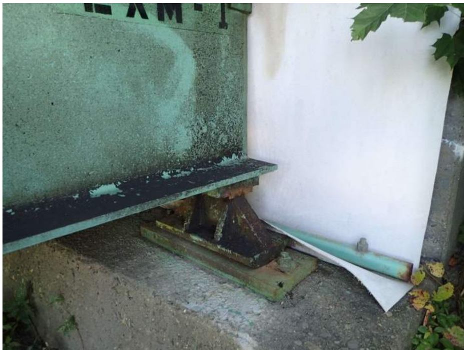
PHOTO 48 Condition Description Abutment 1 - Girder 1 rocker bearing (60 F)
