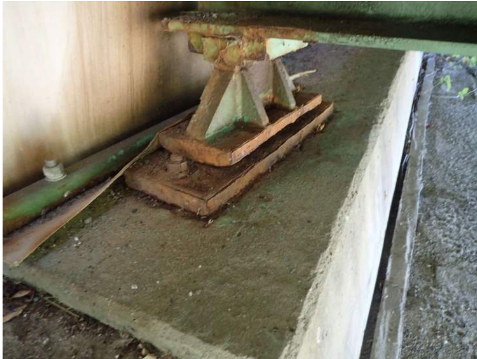
PHOTO 43 Condition Description Abutment 1 - Girder 3 rocker bearing (60 F)
