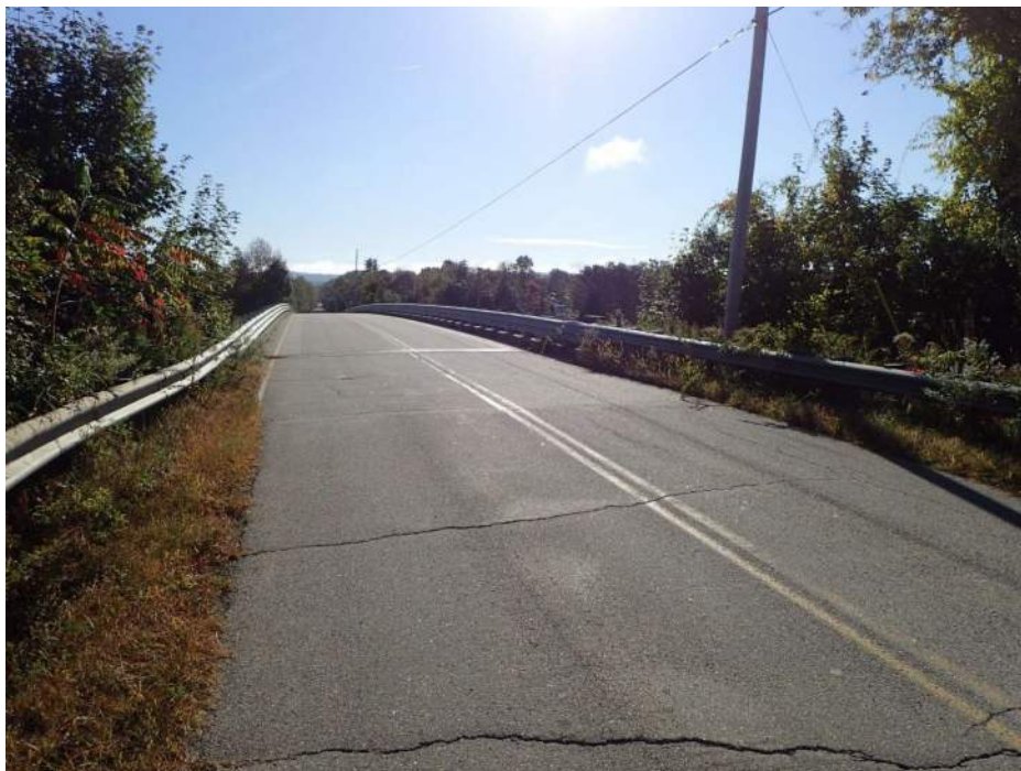
PHOTO 6 Condition Description West Approach - Wide cracking in pavement
