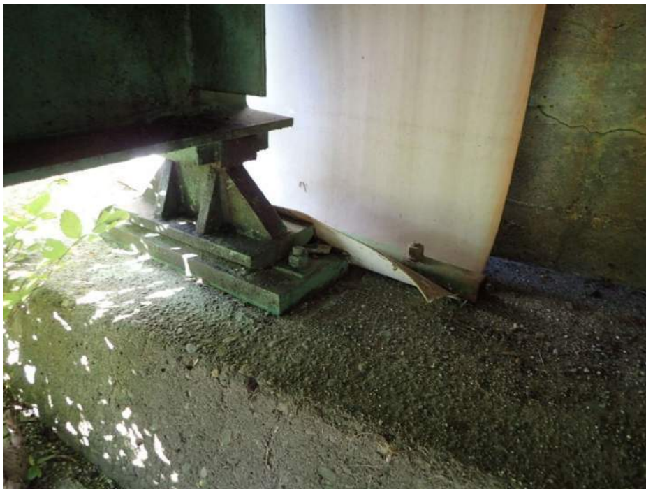
PHOTO 41 Condition Description Abutment 1 - Girder 4 rocker bearing (60 F)
