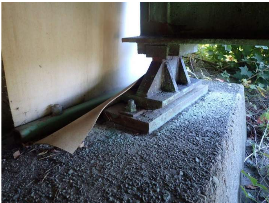
PHOTO 47 Condition Description Abutment 1 - Girder 1 rocker bearing (60 F)
