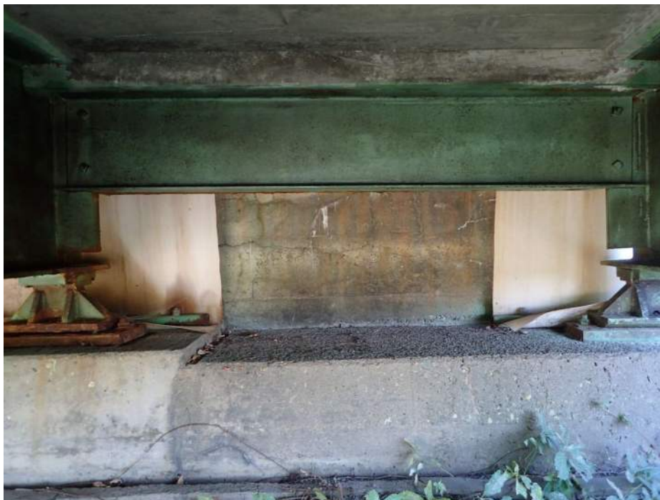
PHOTO 46 Condition Description Abutment 1 - bay 1, girders 2 & 1, moderate cracking on backwall
