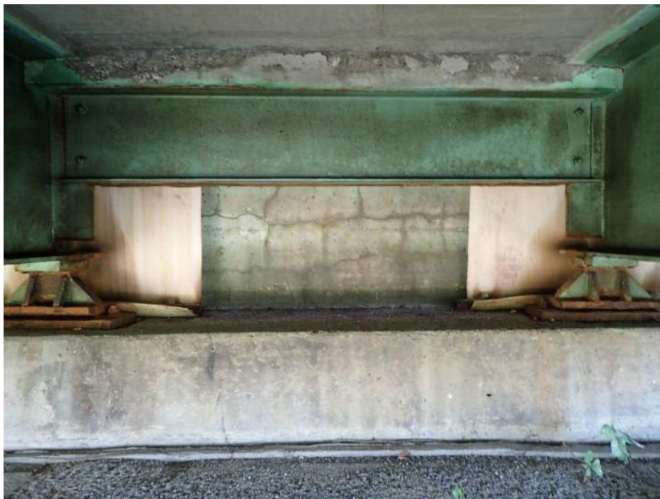
PHOTO 44 Condition Description Abutment 1 - bay 2, girders 3 & 2, moderate cracking on backwall
