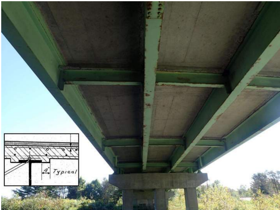
PHOTO 62 Condition Description Span 2 - deck & framing looking East & typical haunch detail.
