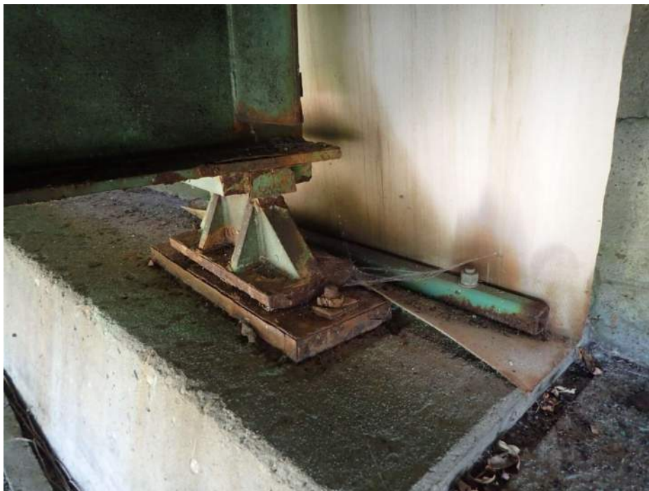
PHOTO 45 Condition Description Abutment 1 - Girder 2 rocker bearing (60 F)
