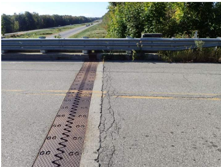
PHOTO 8 Condition Description Finger Joint over Abutment 1 - looking South, heavy map cracking before backwall
