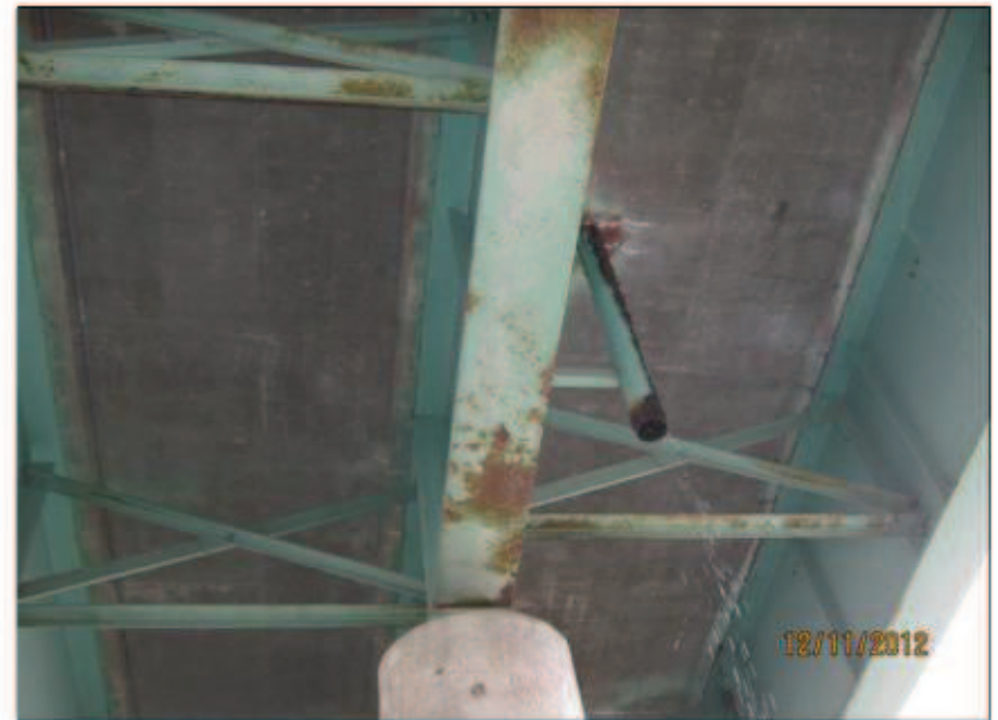
Girder/drain – rust is worst case
