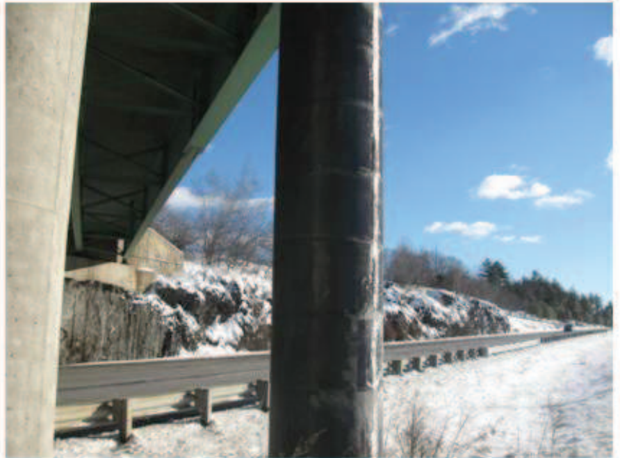
Wrapped east pier column
