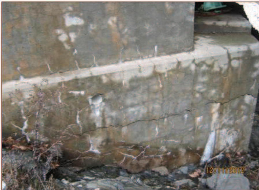
Northerly wing/seat - note heavy cracking
