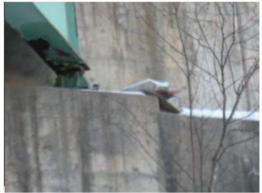
Debris on bridge seat south abutment
