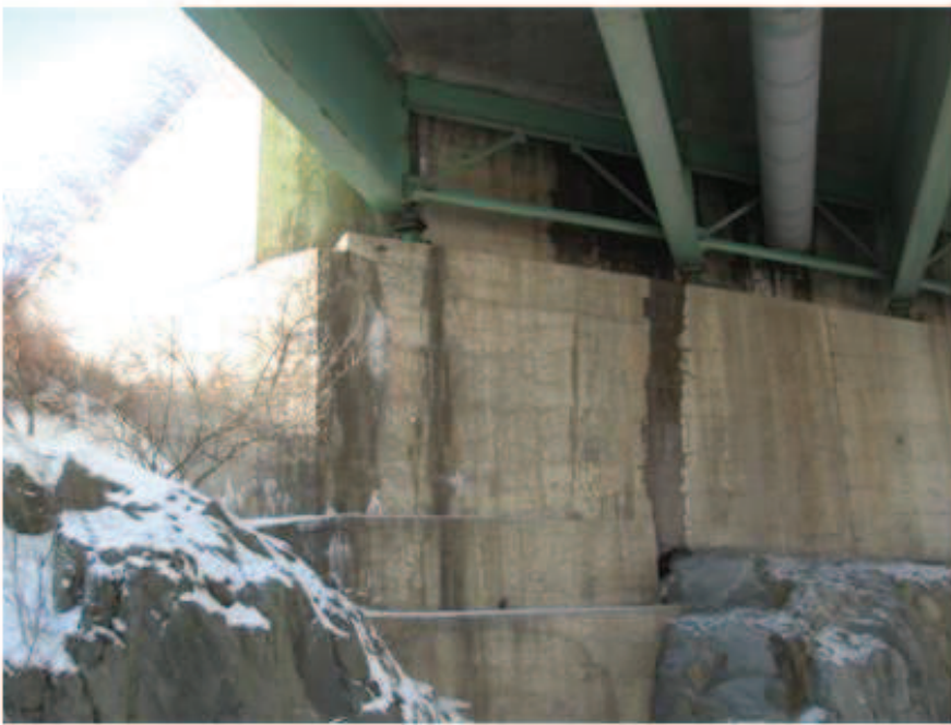
Heavy cracking & staining at SE wing turn
