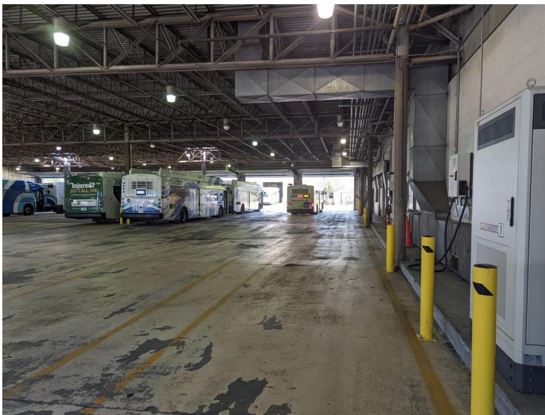
**Figure 5 Existing DC Fast Chargers at 114 Valley St Facility**
