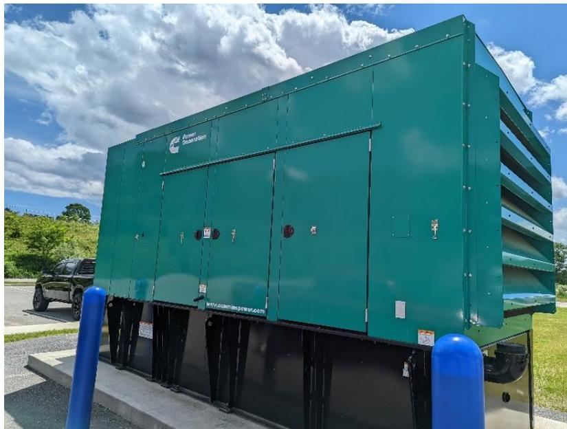
**Figure 12 Existing Diesel Generator Providing Power to the Depot During Outages**
