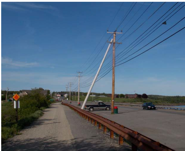
Photo 1. Route 1 Causeway with parking, Downeast Sunrise Trail/Rail Corridor.
