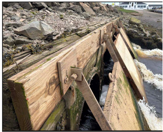
Photo 2. Dike Bridge culverts with flap gates downstream.
