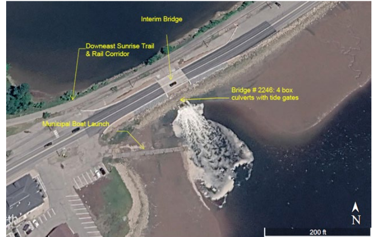
Photo 4. Aerial view of Interim Bridge Location
