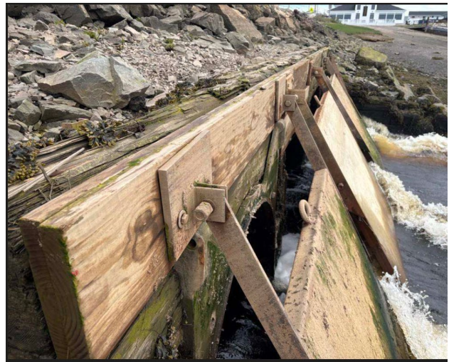
Photo 2. Dike Bridge culverts with flap gates downstream.
