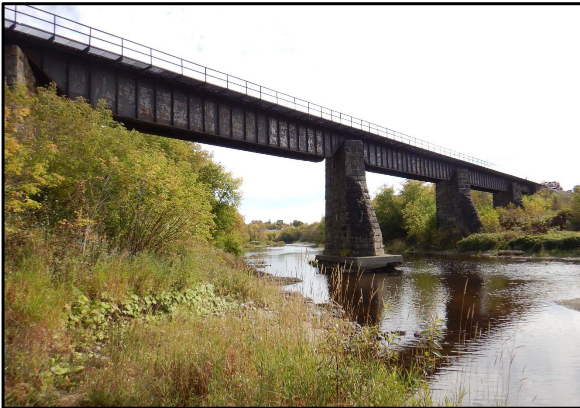
Elevation View of Bridge Looking South
