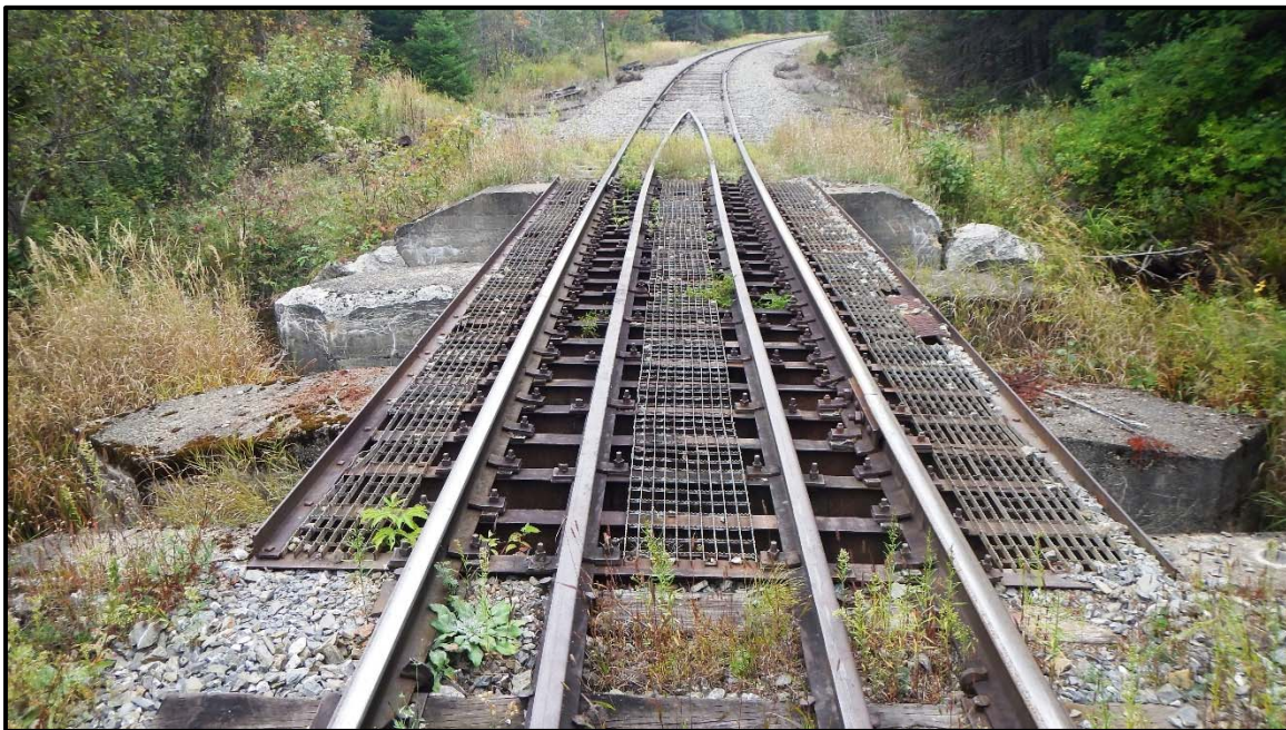
View on Centerline of Bridge Looking Northeast
