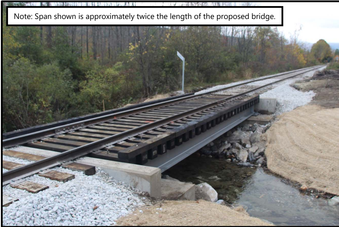
2014 Replacement Steel Girder on Precast Concrete Substructure on Vermont Railway (VTR) – Dorset, VT
