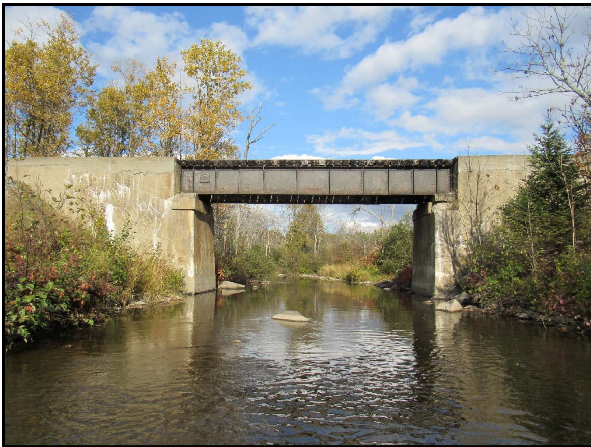
Elevation View of Bridge Looking East
