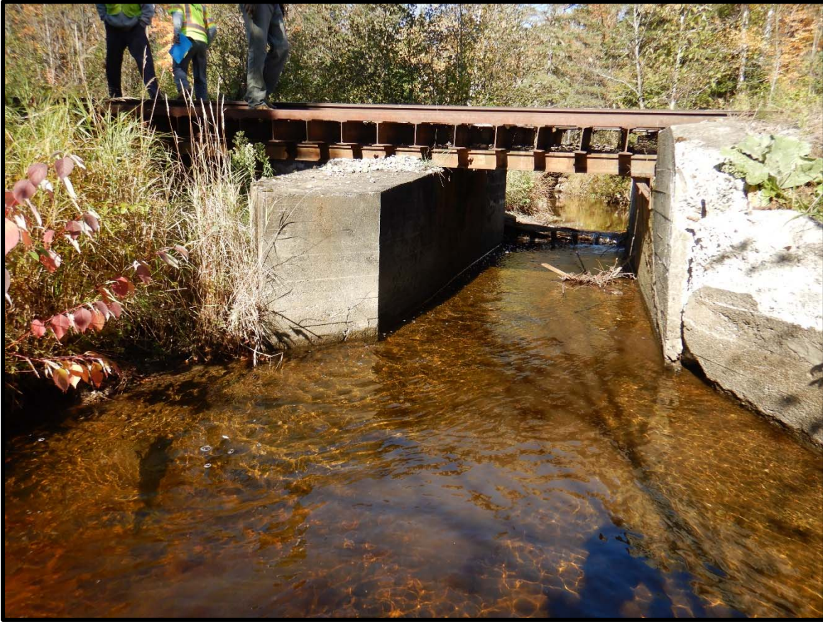
View of Northeast Wingwall, North Abutment and Pier Looking West
