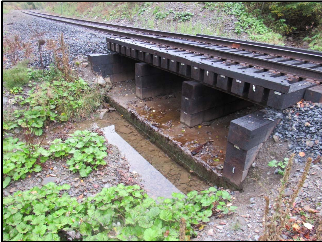
2014 Replacement "Rail-top" Superstructure on Madawaska Subdivision (Br. 7791 MP251.75)
