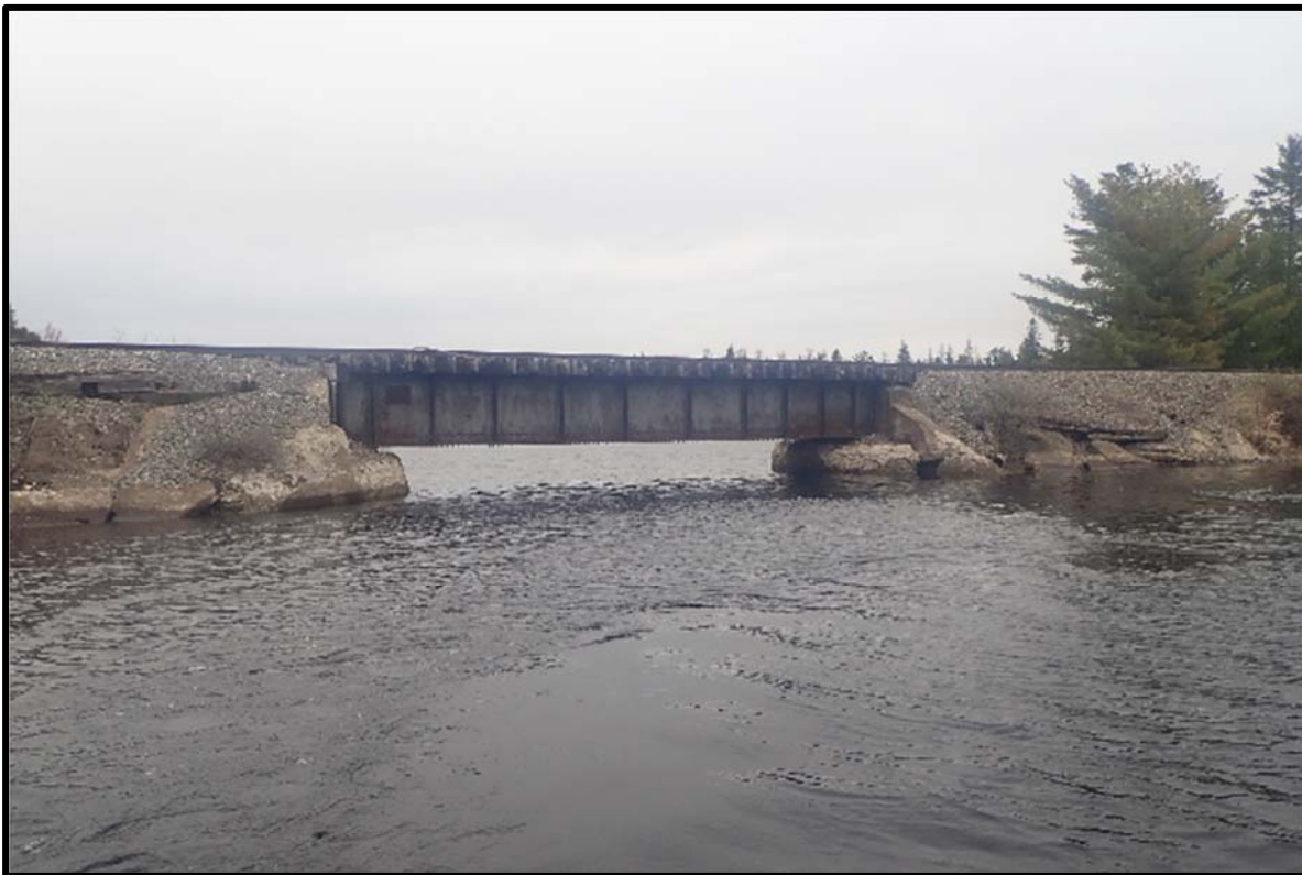
Elevation View of Bridge Looking North
