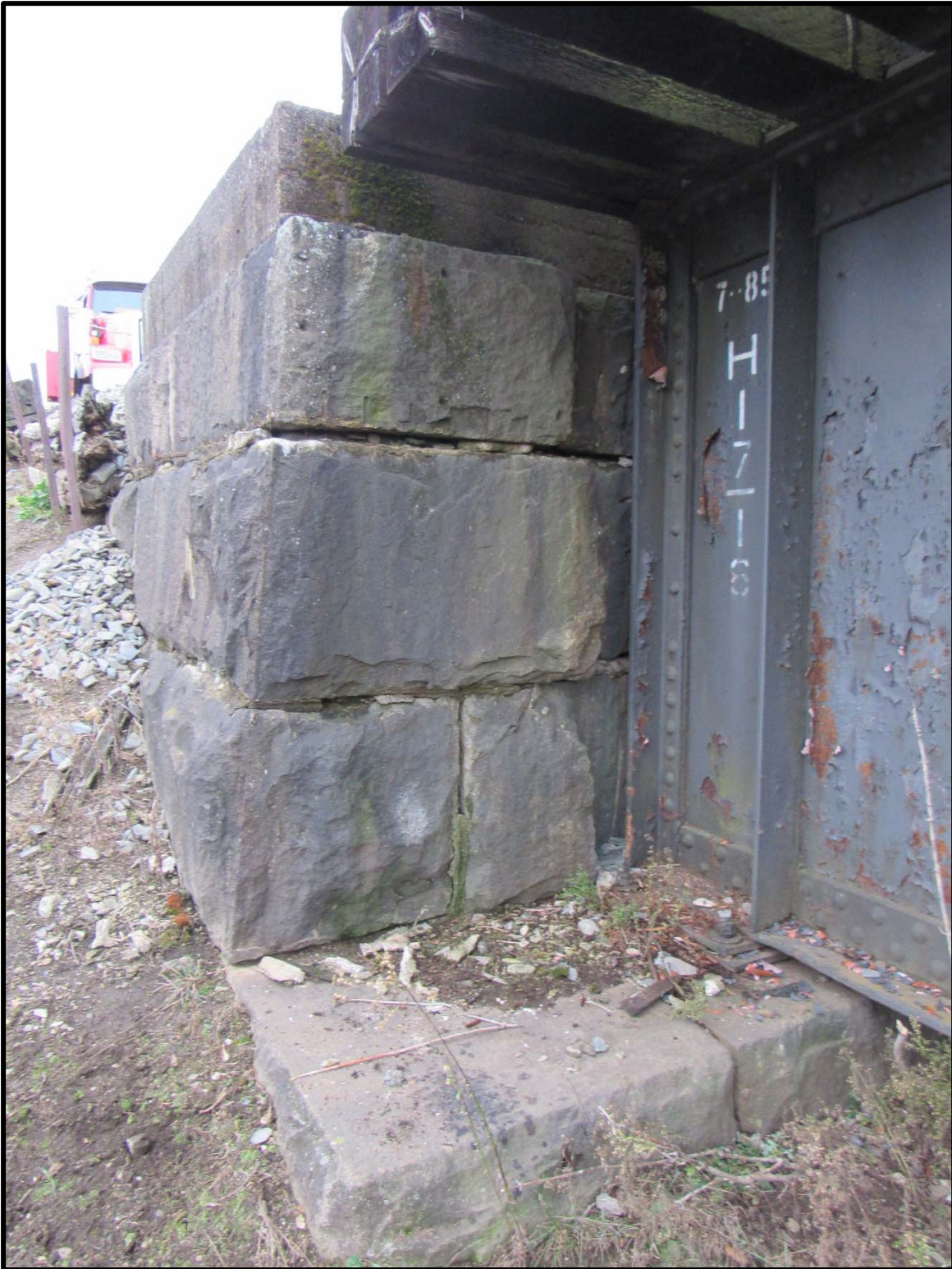
East End of South Abutment
