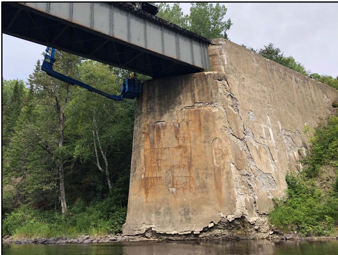
View of North Abutment and Northeast Wingwall
