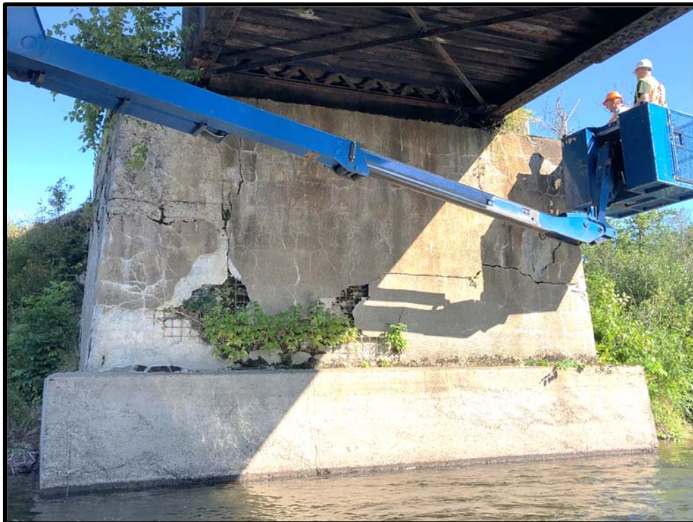
View of North Abutment
