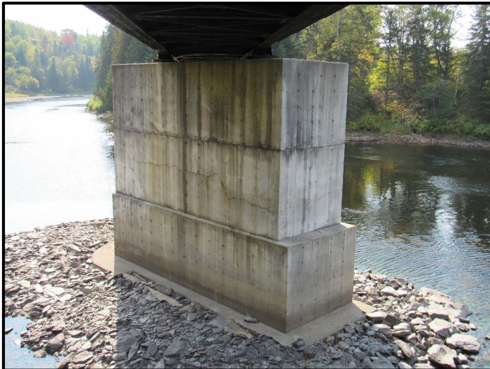
North Elevation of North Pier, South Pier Similar (Encased in 2008)
