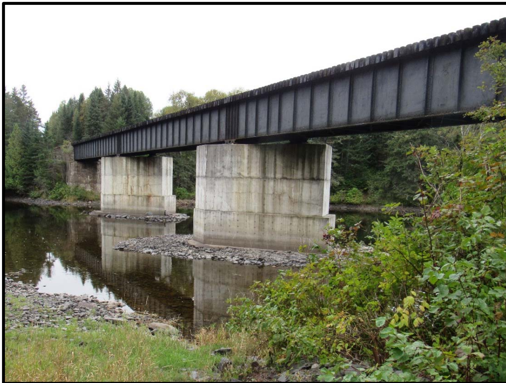
Elevation View of Bridge Looking Southwest
