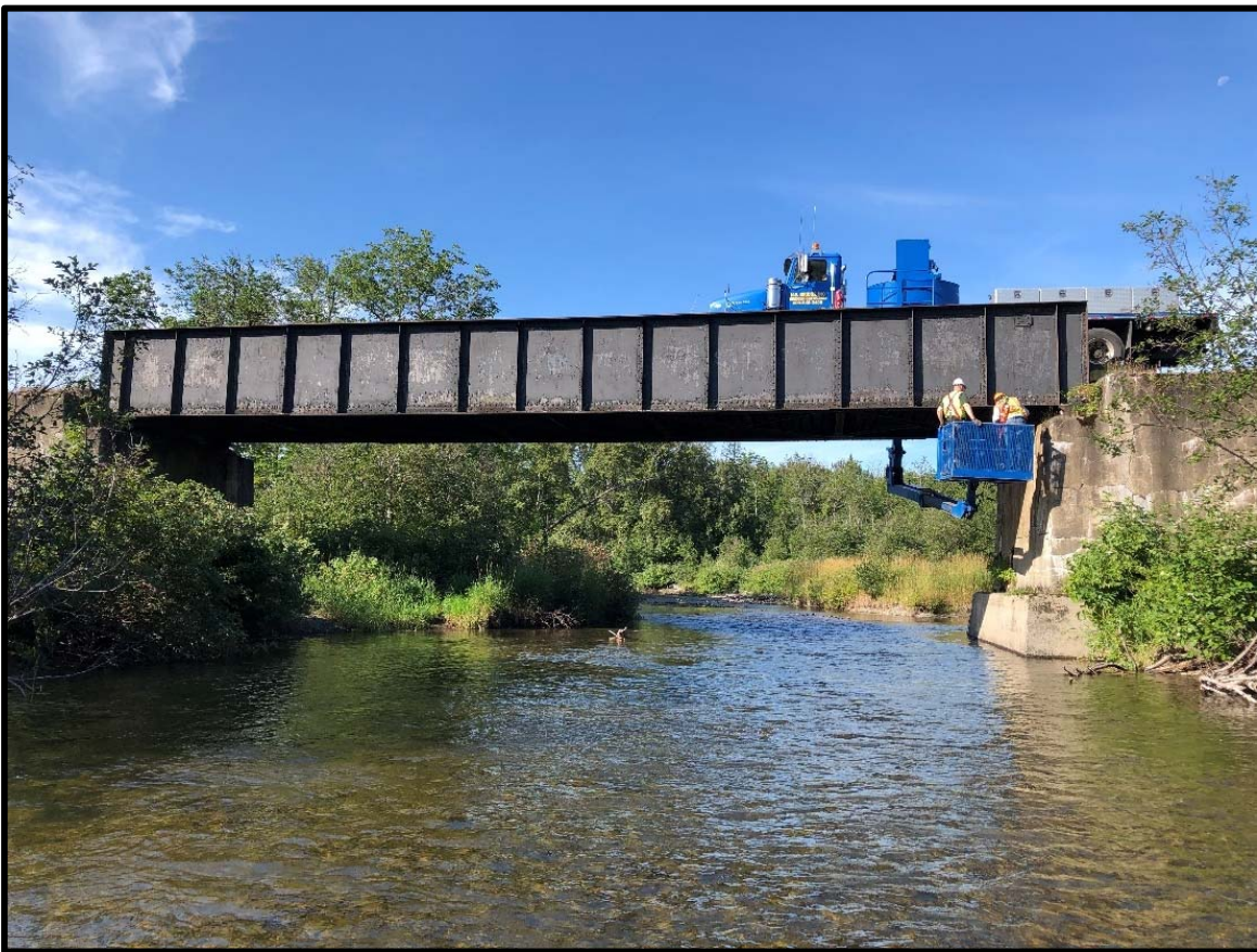
Elevation View of Bridge Looking West
