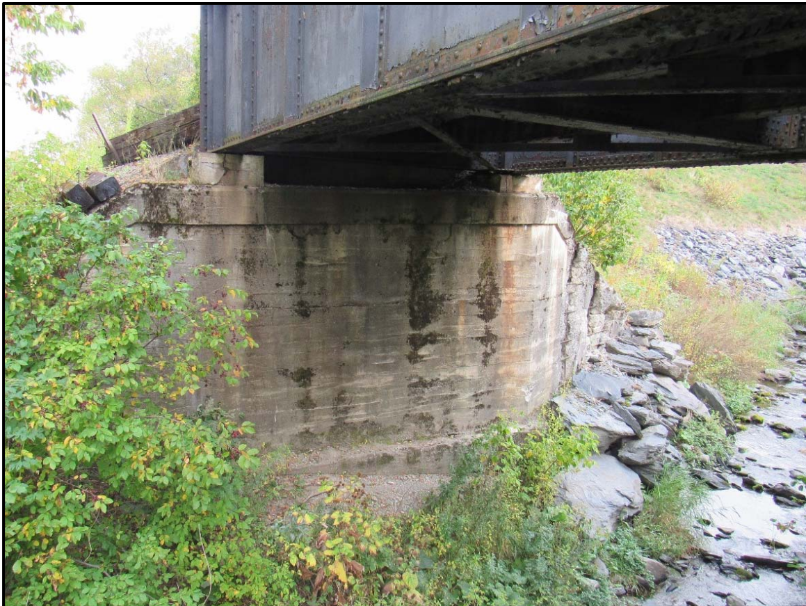
Elevation View of North Abutment
