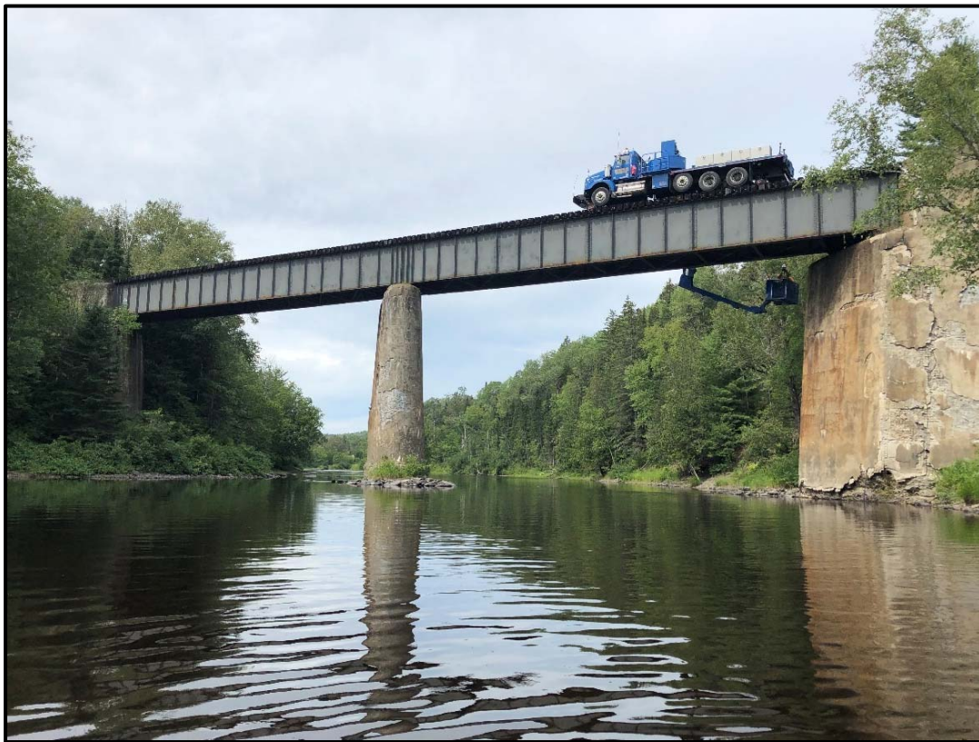
Elevation View of Bridge Looking West
