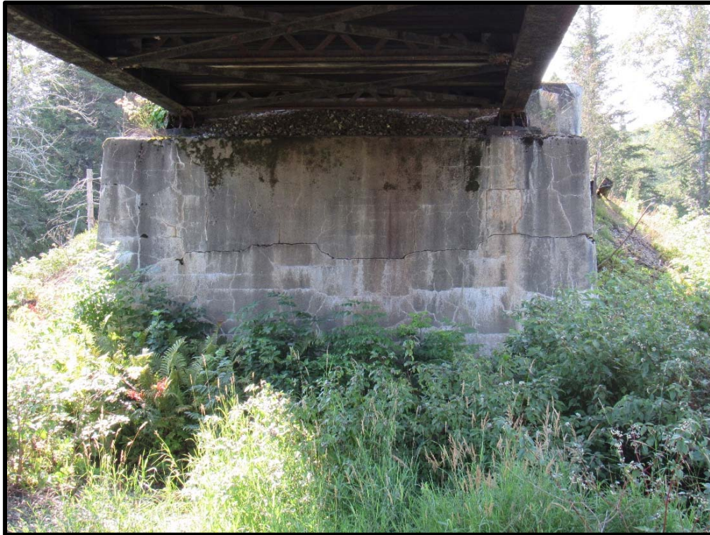
View of South Abutment
