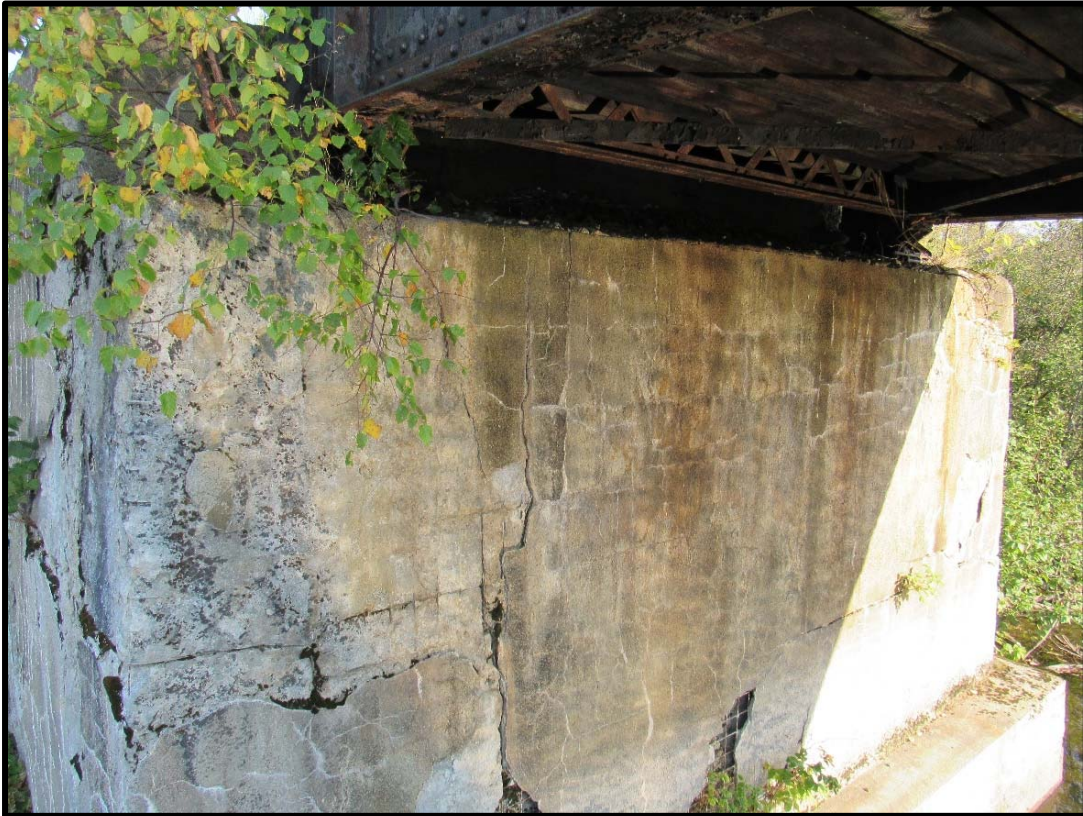
View of North Abutment Bridge Seat and Breast Wall
