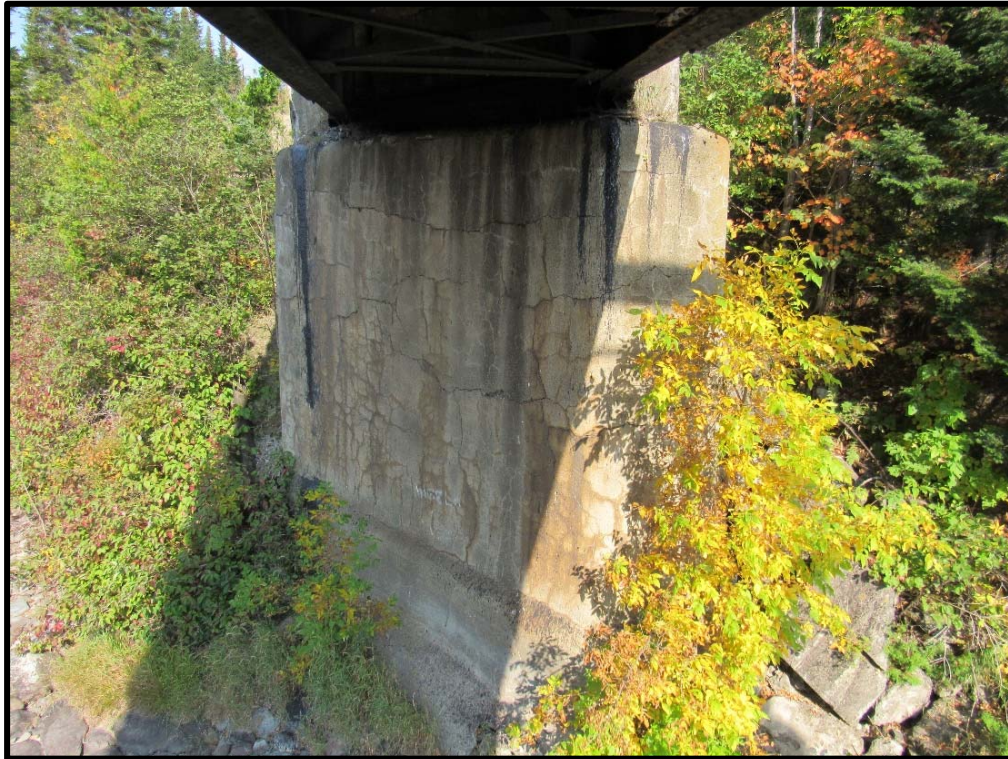
View of North Abutment
