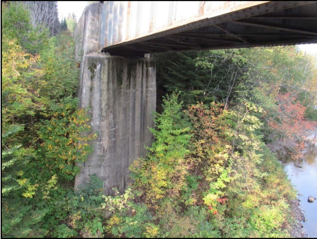
View of South Abutment
