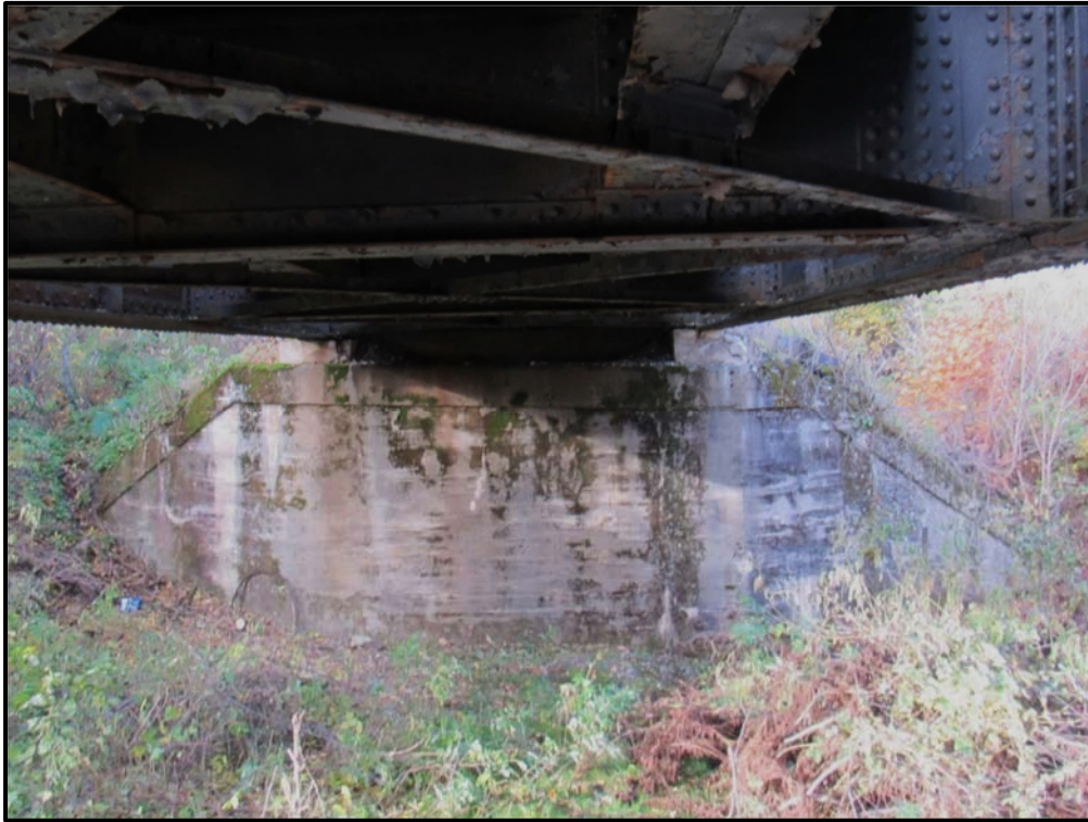
Elevation View of South Abutment
