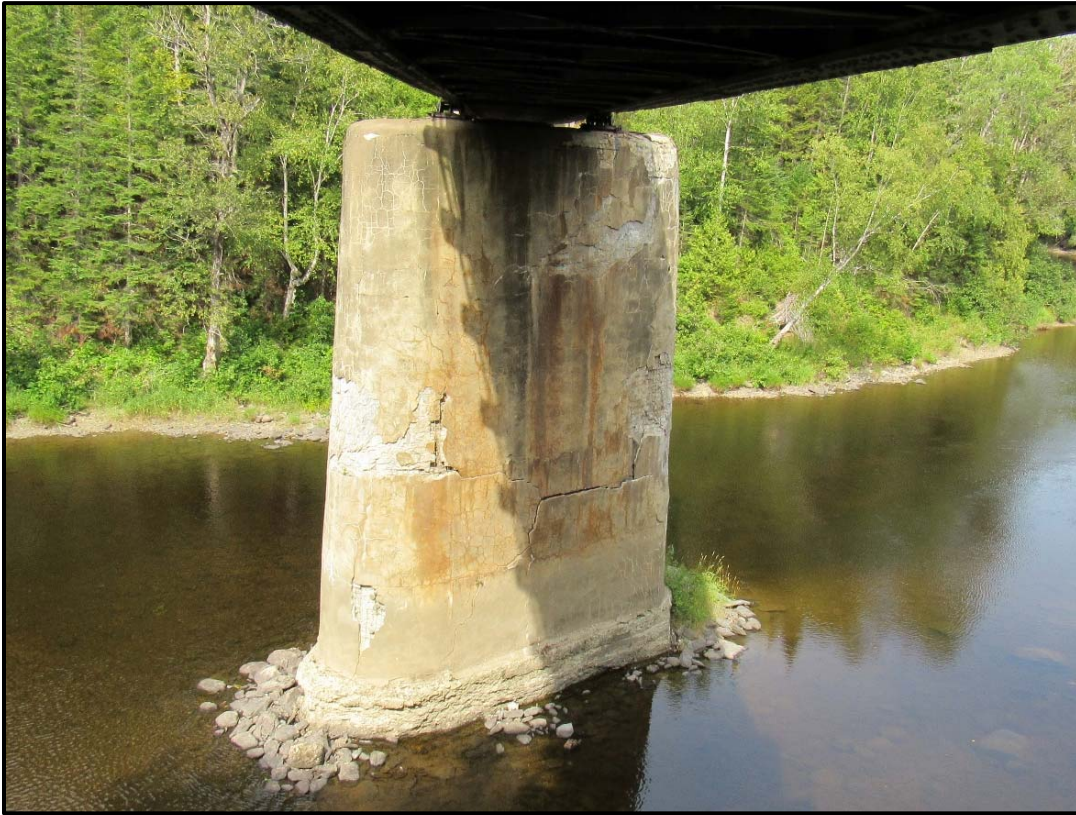
View of South Face of Pier
