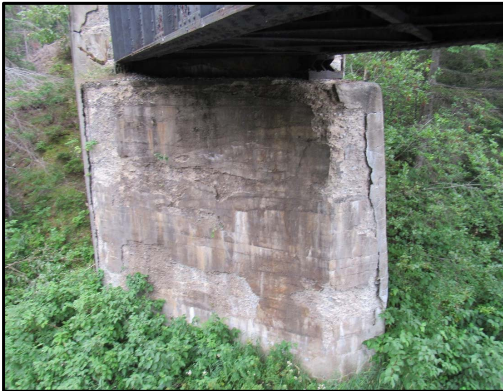
View of South Abutment
