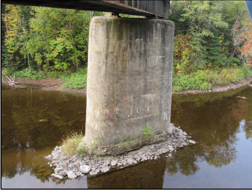
North Face of Pier (Encased in Shotcrete)
