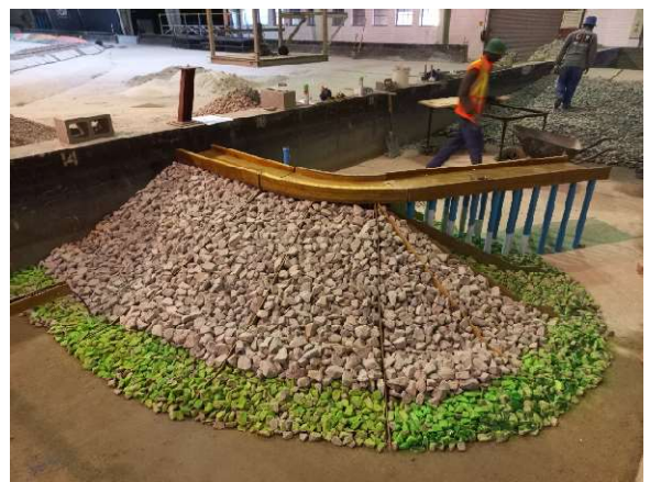
Placement and shaping of model armour rock. The wooden capping was also completed and fitted to the rubble mound breakwater and vertical piles.
