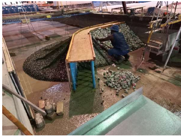
Dismantling the test structure after completion of Test Series A, and reconstructing different rock for the underlayer and armour layer.
