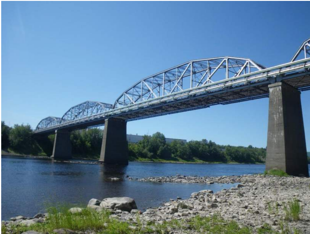
Photo 1: East Elevation, Looking Southwest. Note paper process pipes for the Twin Rivers Paper Company along east truss, cracks with efflorescence in pierwalls and rock aggradation along embankment.
