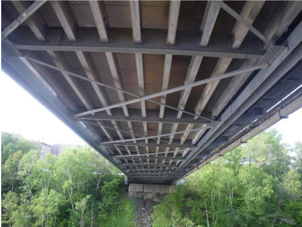
Photo 9: Underside of Span 4 near Pier 3, Looking South.
