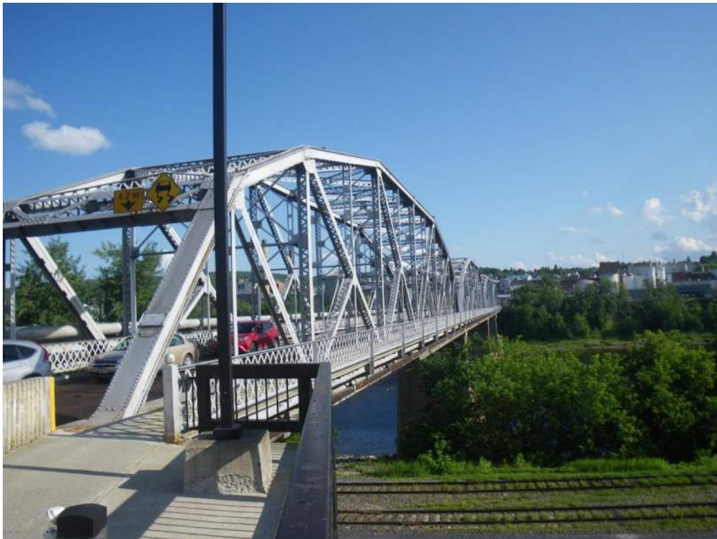
Photo 2: West Elevation, Looking South. Note span 1 over railroad tracks, "At-Bridge" vertical clearance sign and conduits/abandoned pipe along west truss.
