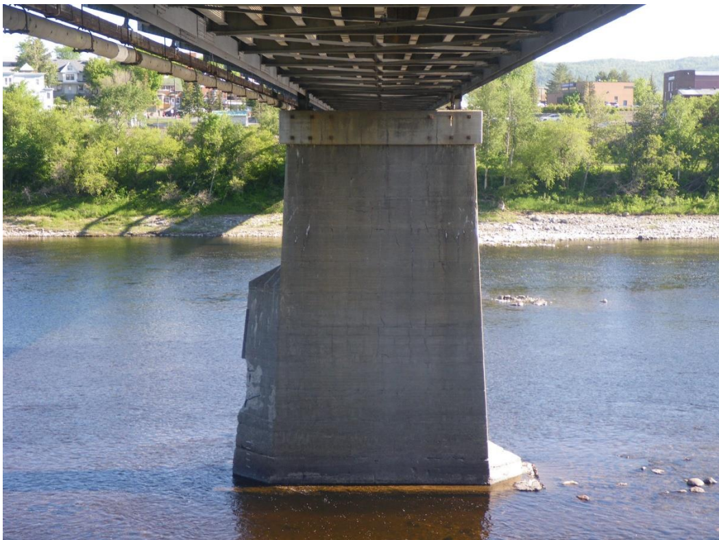
Photo 10: Pier 3, South Face. Note steel post-tensioning rods in pier cap.
