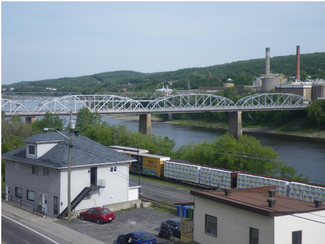
Photo 2: West Elevation, Looking Southeast. Note span 1 over CN railroad tracks.
