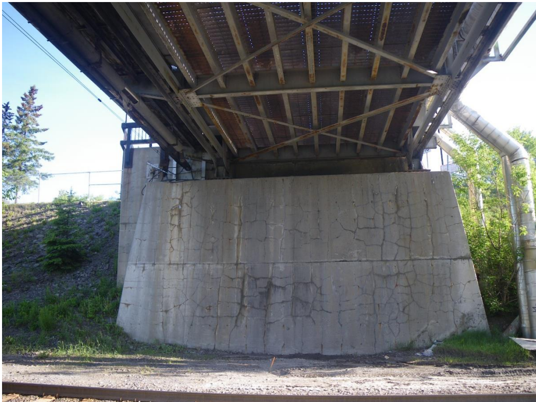
Photo 8: North Abutment, Looking North.
