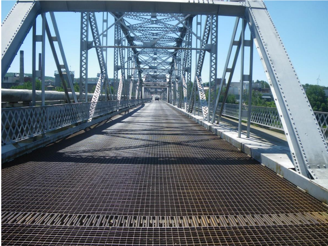
Photo 5: Typical Top of Deck near Pier 1, Looking South into Span 2.
