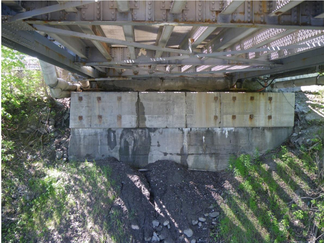
Photo 9: South Abutment, Looking South. Note bridge seat with steel post-tensioning rods.
