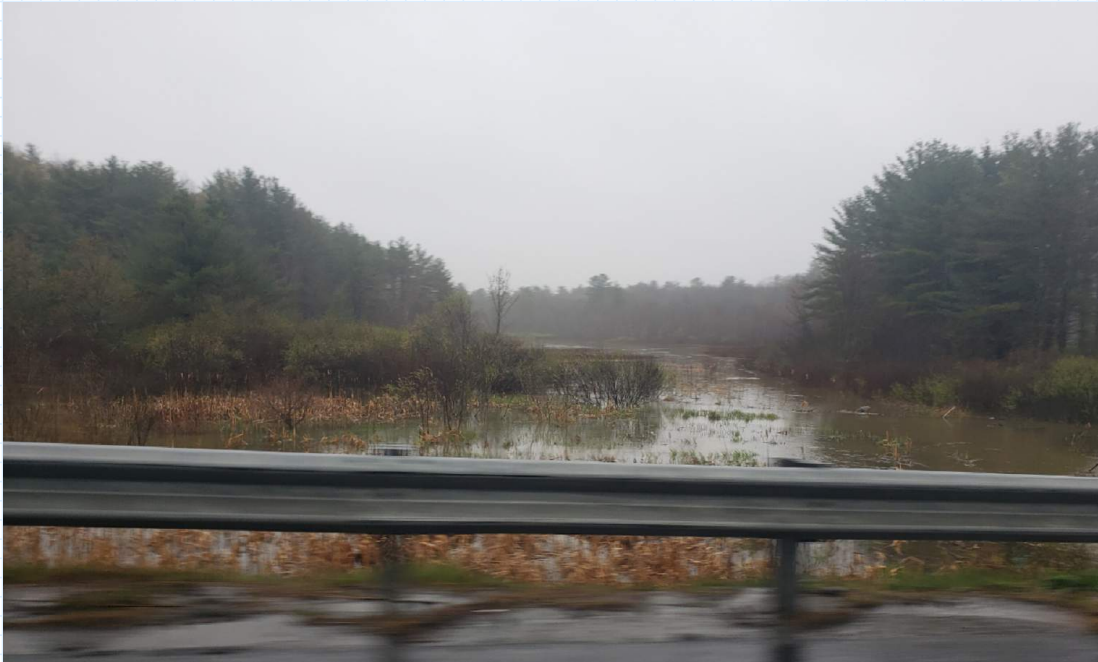
May 1, 2023 Storm - MaineDOT Photo - Downstream, Beaver dam submerged
