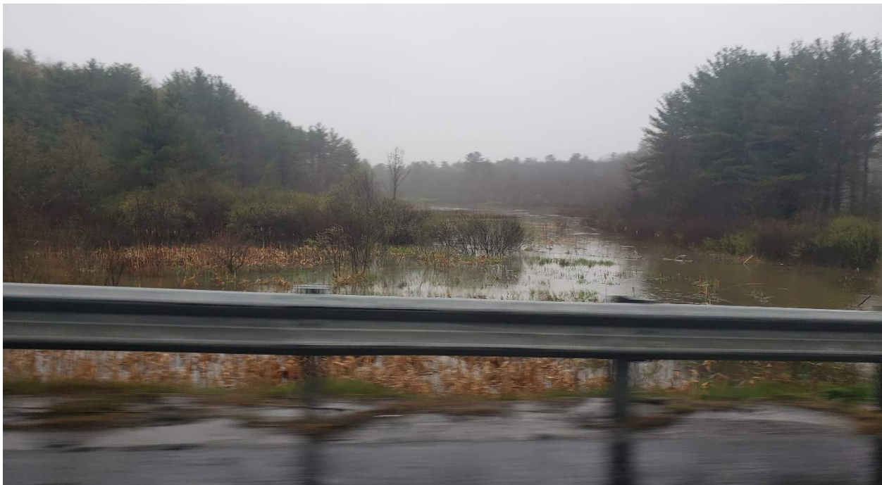
Figure 3: Downstream of Thorne Brook Bridge after a storm (5/1/2023)
