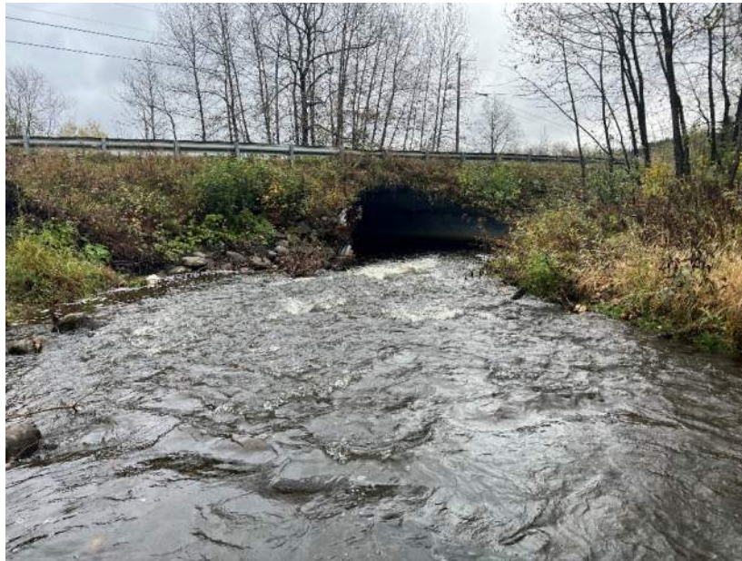
Photo 5: View of downstream bridge section from right bank.
