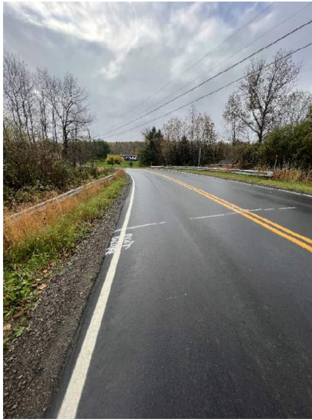
Photo 1: Approach roadway looking southeast towards Bridge No. 5309.
