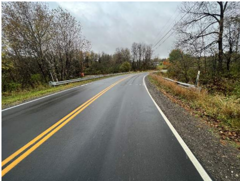
Photo 4: View of approach roadway looking north.
