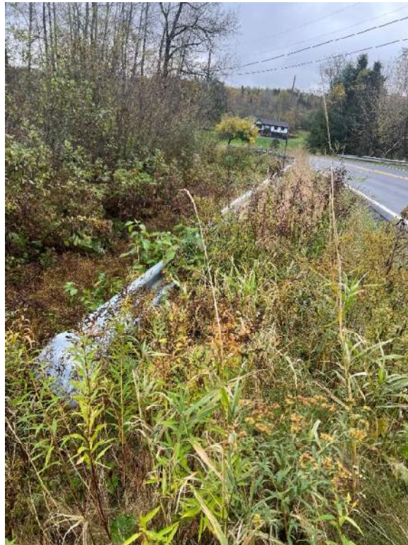
Photo 8: Looking southeast at guiderail on top of bridge.
