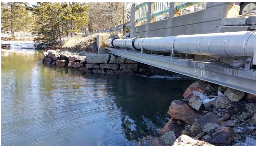
Figure 15. Upstream face mid-falling tide. Note utility line near upstream face of bridge.
