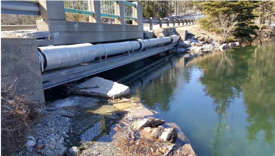
Figure 3. Upstream face of bridge near high tide. Utility line is lower than existing low chord.
