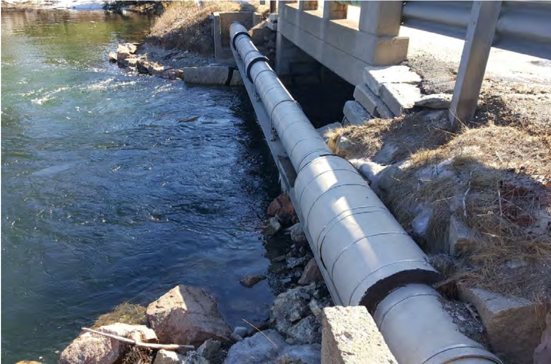
Figure 29. Utility line just upstream of existing bridge.
