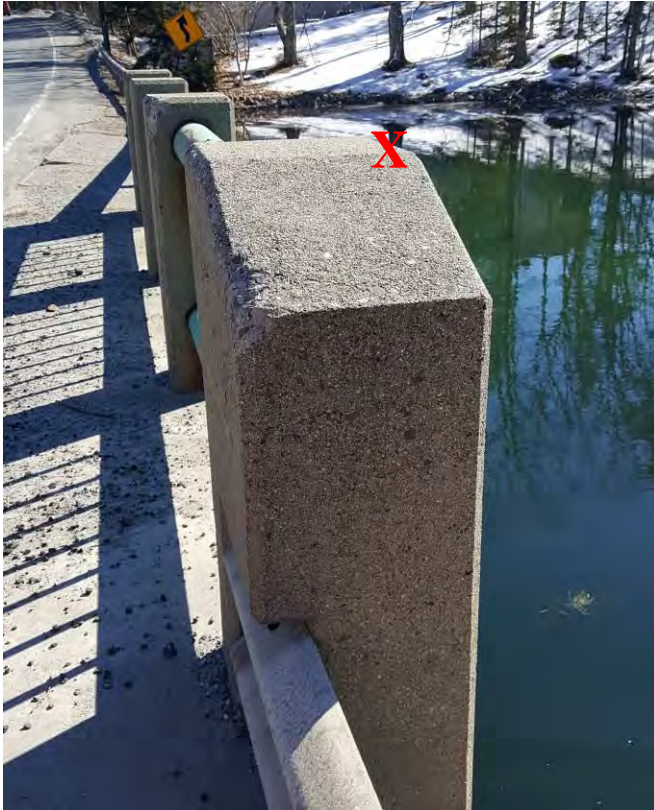
Figure 12. Example tide measurement location from top of rail at DS Right Abutment (red X).
