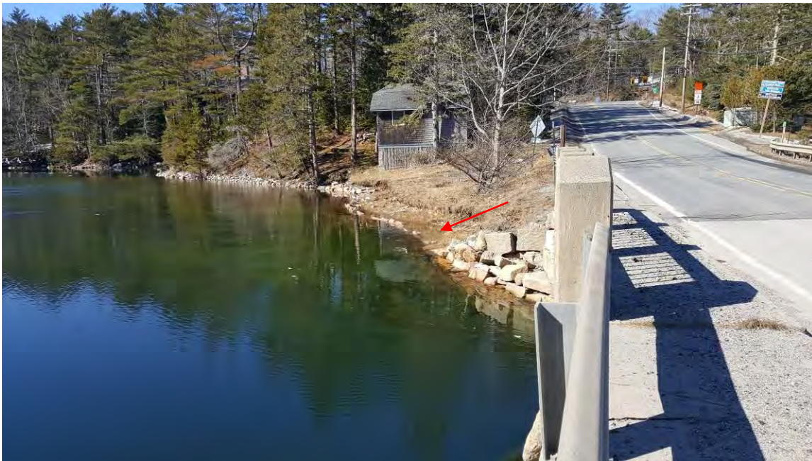
Figure 32. Westerly downstream embankment location of piping (red arrow)
