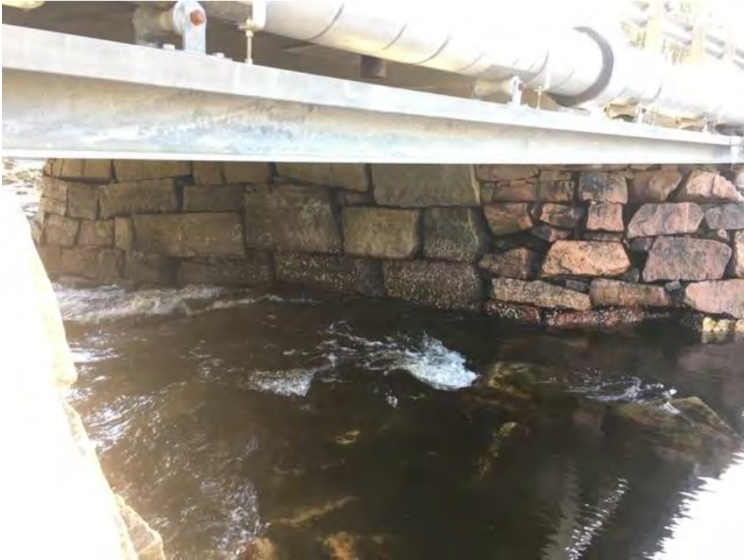
Figure 16: Looking at west abutment at mid-falling tide, note grade control in channel.
