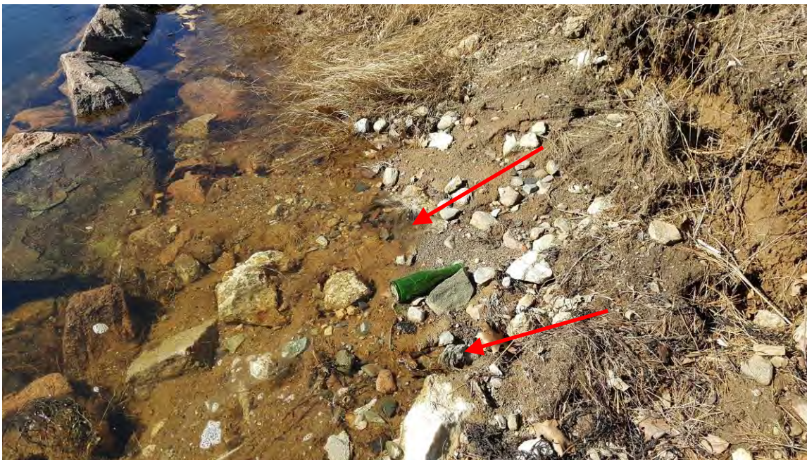
Figure 33. Areas of active piping through embankment, flow from downstream to upstream on incoming tide.
