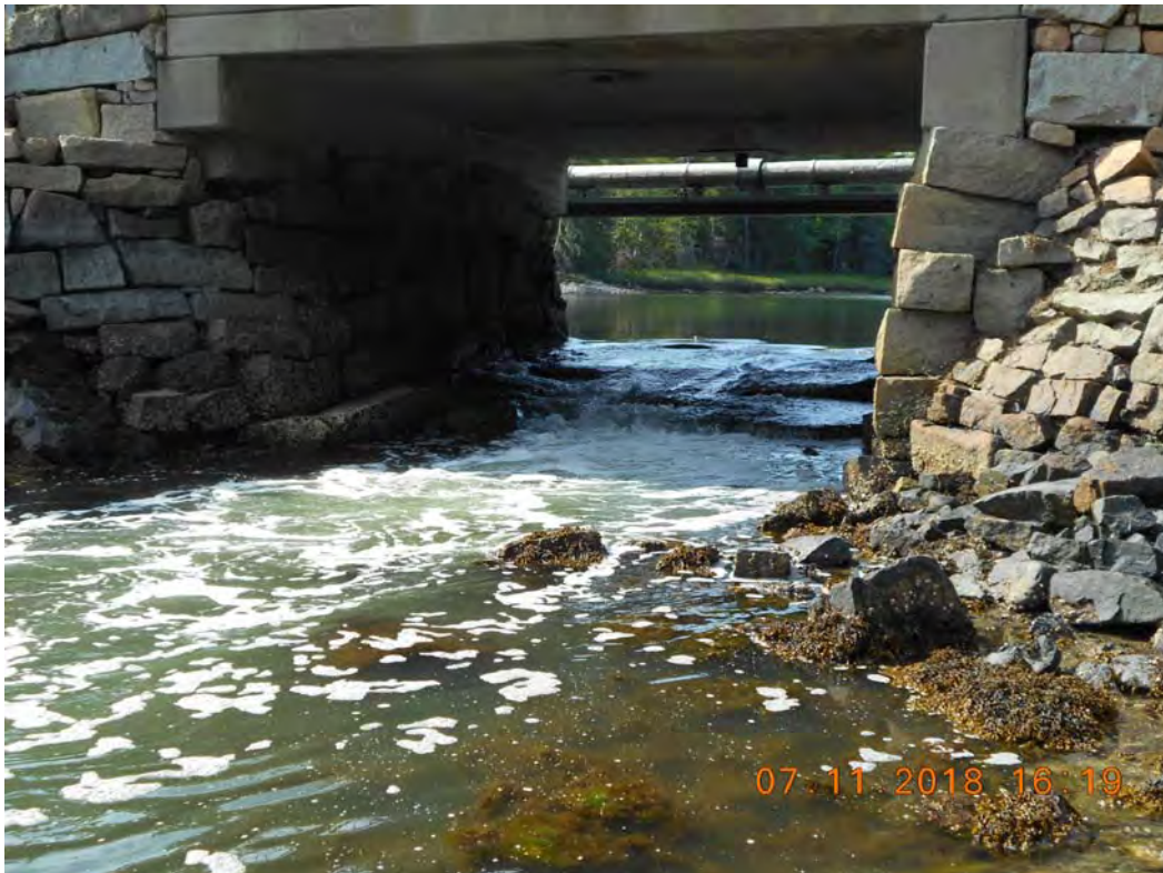
Figure 3. Grade Control at Bridge
