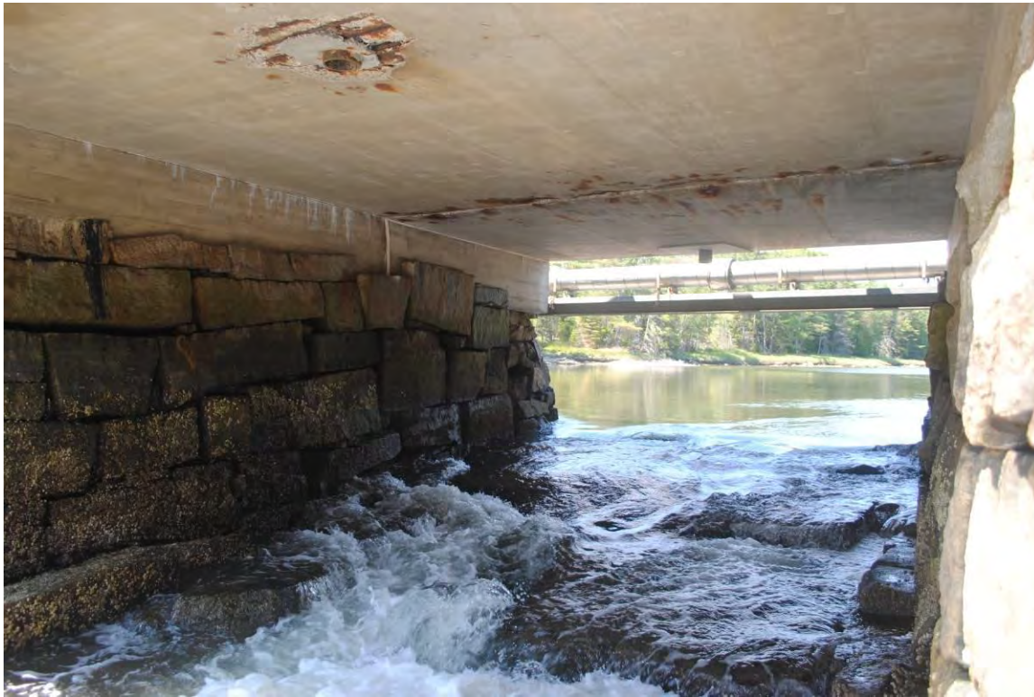
Figure 30. Photo looking upstream into the bridge showing bed protection. This protection only extends across the existing channel.
