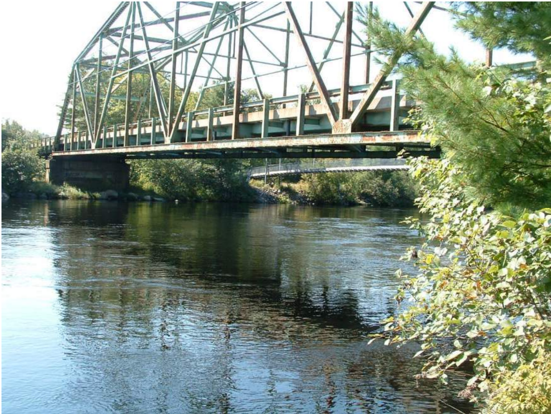
Photo 1 – Existing Structure– Looking Upstream
