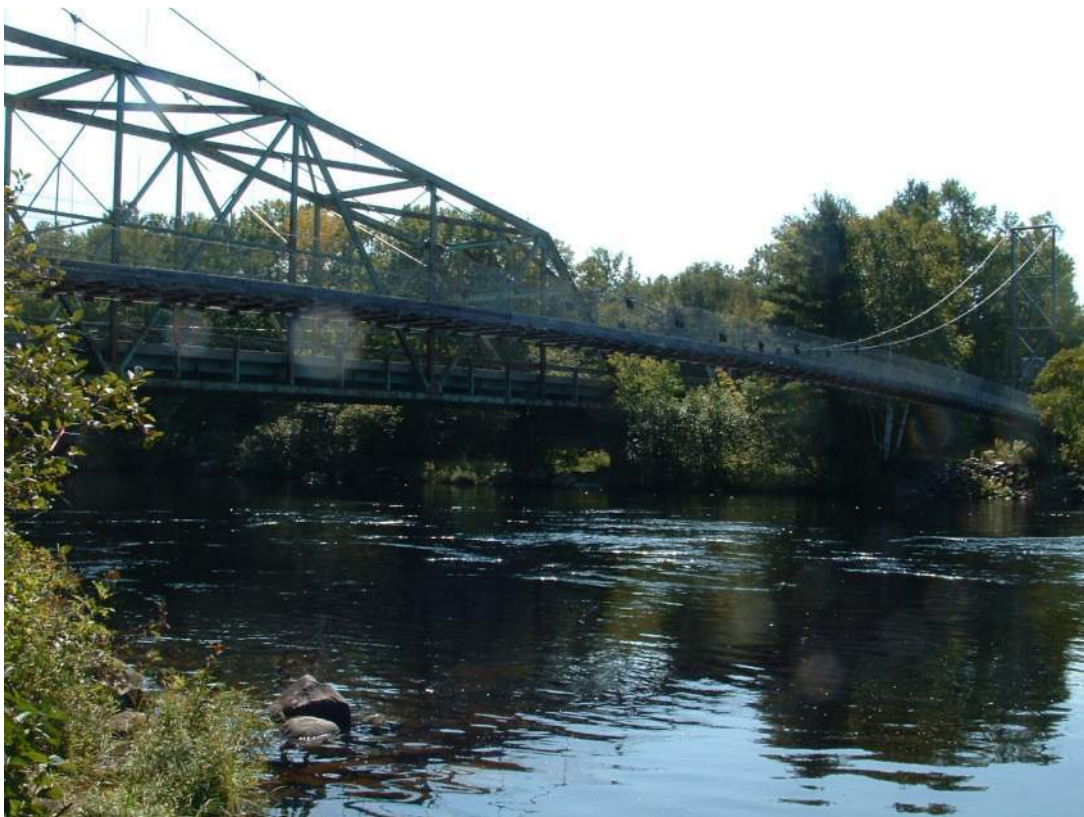
Photo 2 – Existing Structure and Pedestrian Bridge – Looking Downstream
