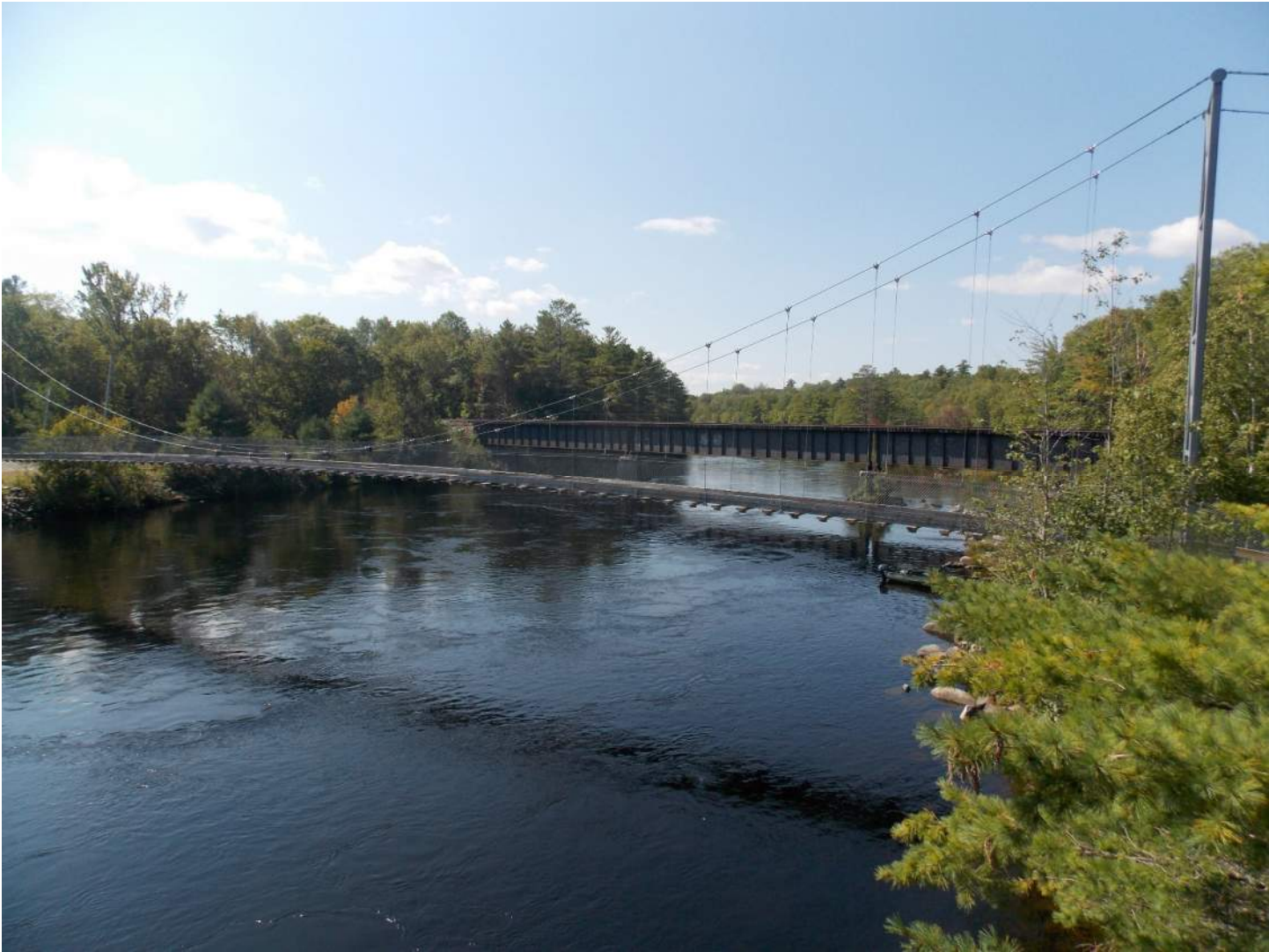
Photo 5 – Upstream Structures – Looking West
