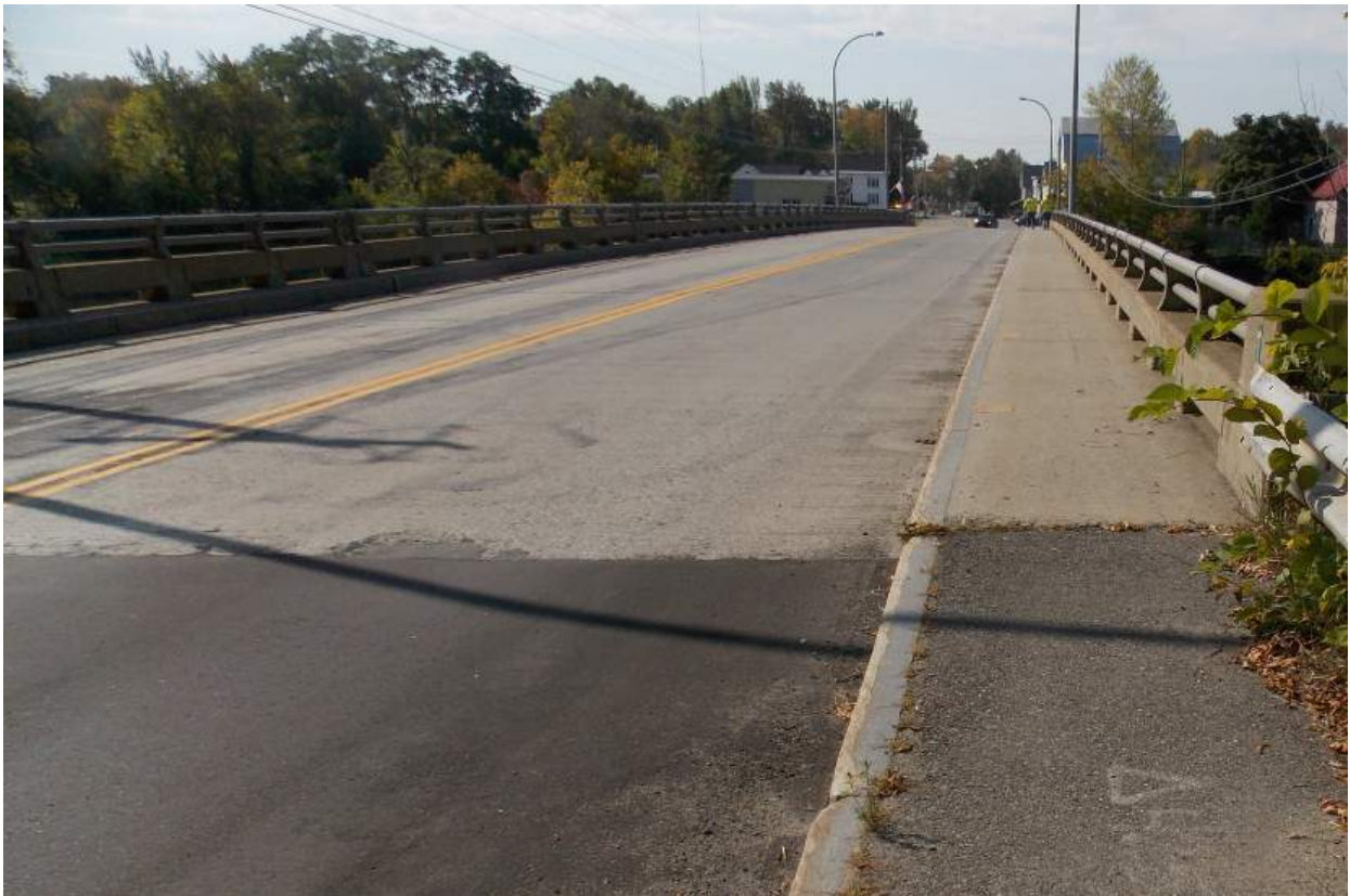
Photo 4 – Main St/ US 2 – Looking South
