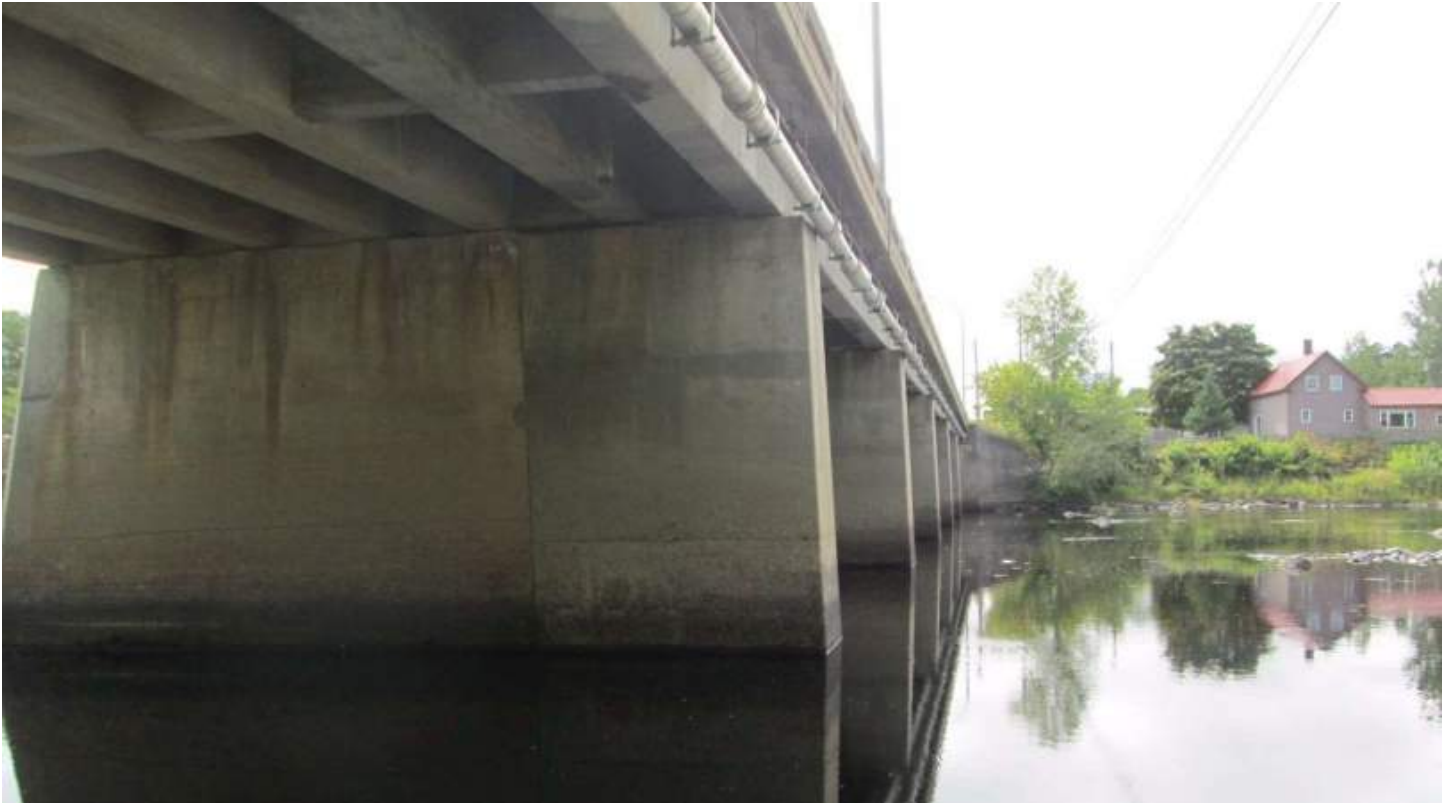
Photo 2 – Western View of Existing Structure – Looking Upstream
