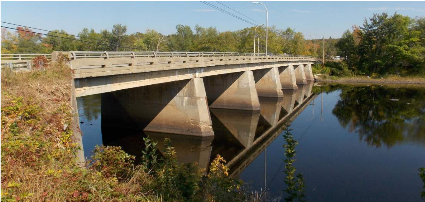
Photo 1 – Eastern View of Existing Structure– Looking Downstream
