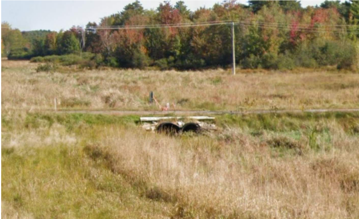
Figure 5: Close-up of posts and rope / chain at private road / driveway from Google Streetview
