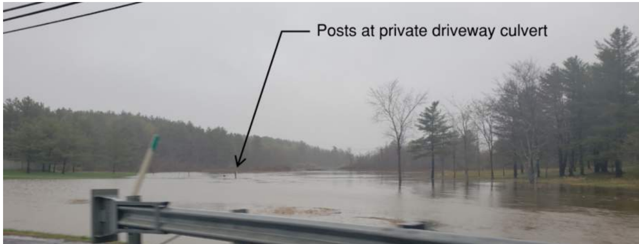
Figure 3: Downstream of Spaulding Brook Bridge during storm (5/1/2023)
