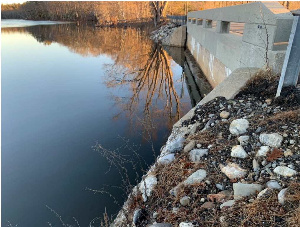
Figure 8. Upstream Water Level After a Rain Event (December 2, 2020)
