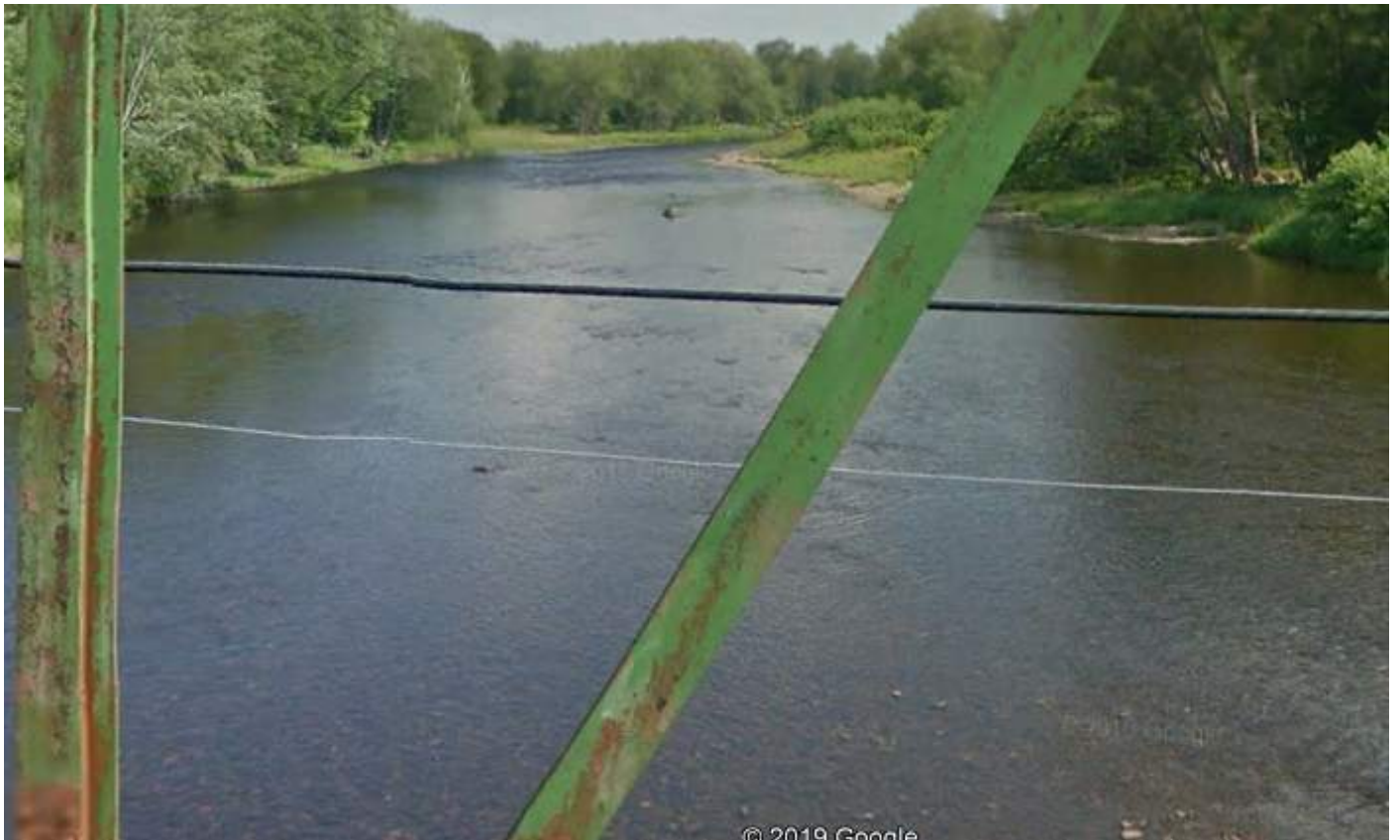
Photo 4 – View of the Downstream Side of Pleasant River – Looking East
