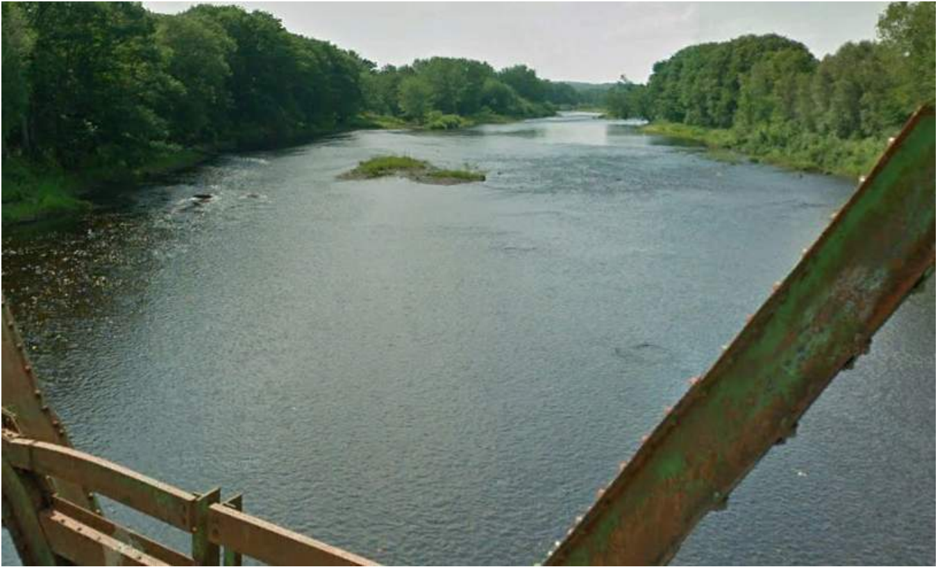
Photo 5 – View of the Upstream Side of Pleasant River – Looking West
