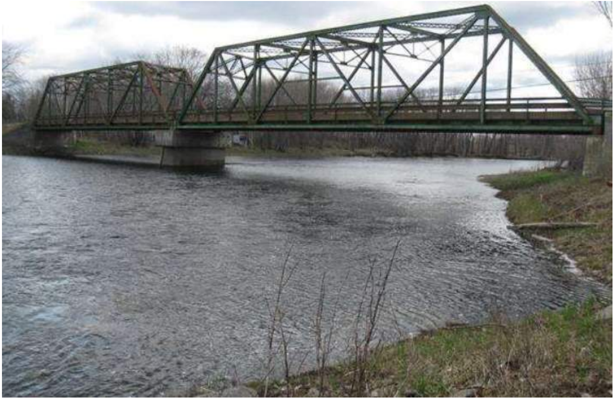
Photo 1 – Eastern View of Existing Structure– Looking Upstream
