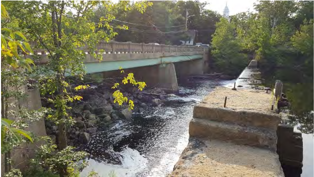
Figure 2 Looking across Dam at upstream face of Bridge.
