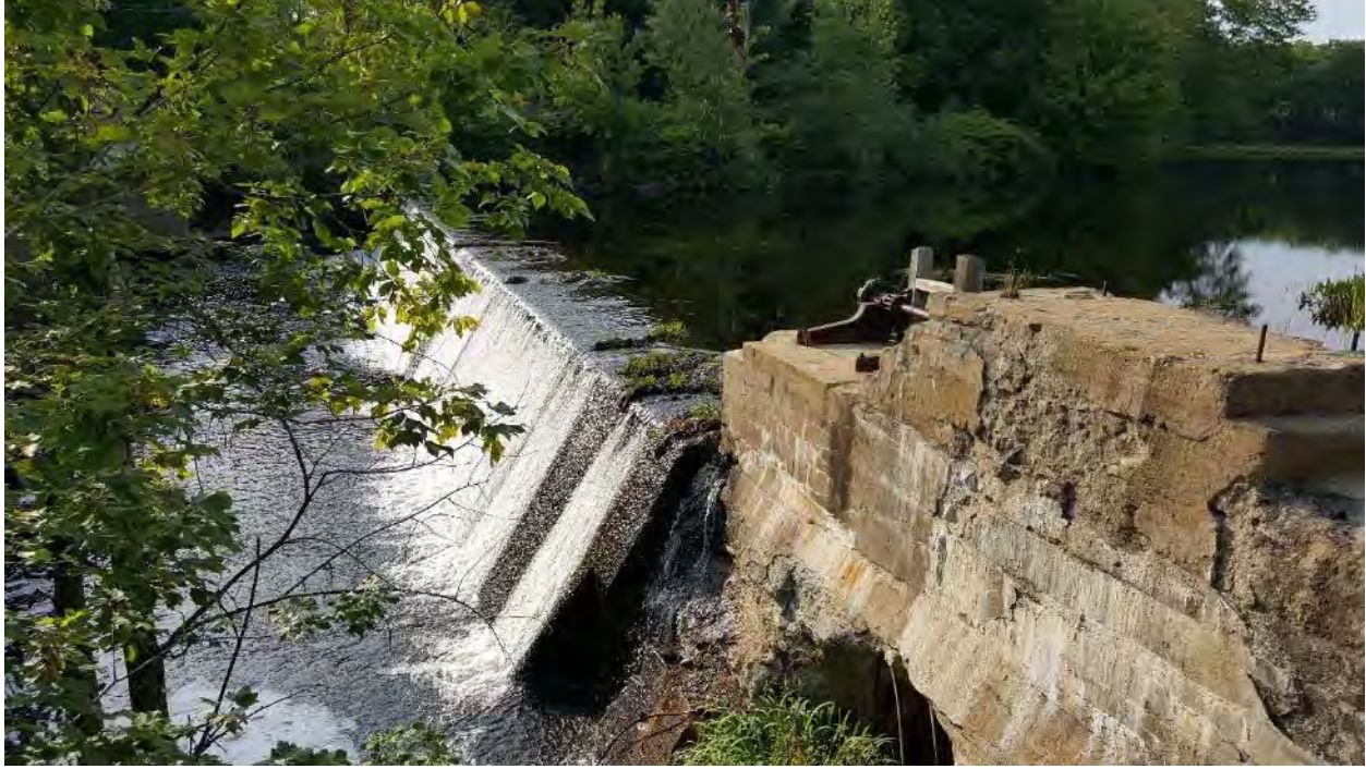
Figure 4 Looking at dam just upstream of bridge
