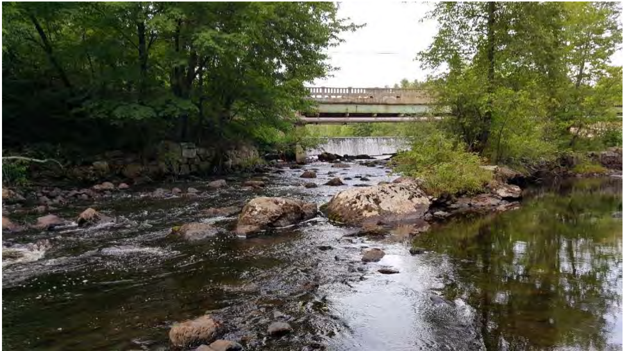
Figure 5 Looking upstream at downstream face of bridge and dam face
