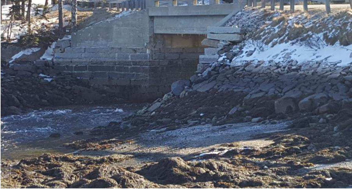
Figure 29. Downstream face of bridge at low tide. Note riprap.
