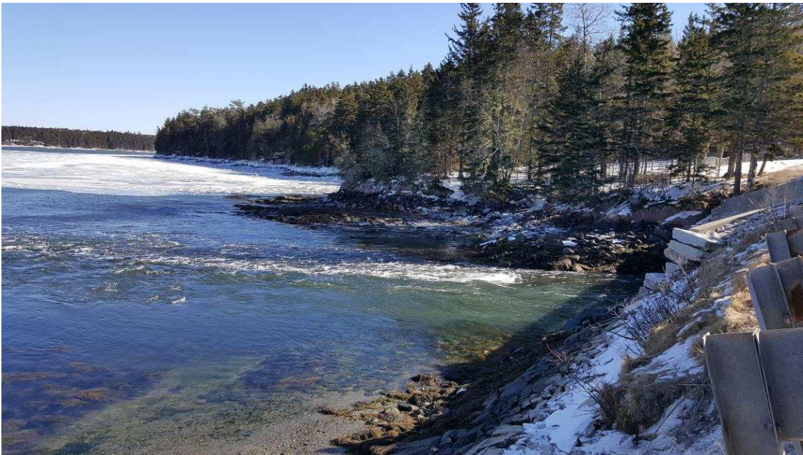
Figure 13. Downstream of bridge, lower tide.
