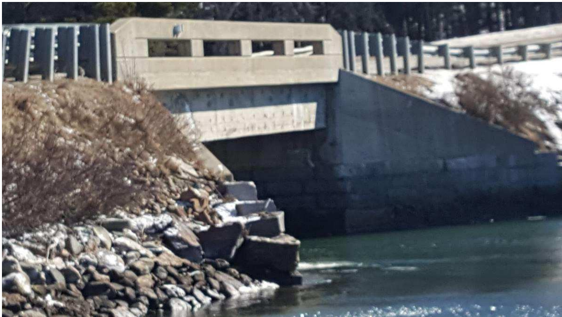
Figure 3. Upstream face of bridge.
