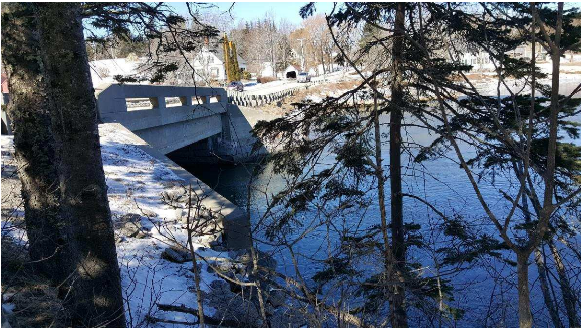
Figure 11. Downstream face, high tide.
