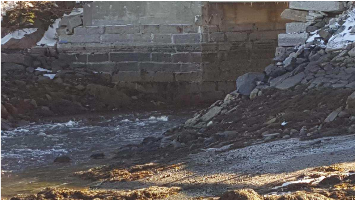
Figure 15. Downstream face. Note tide has dropped below base of bridge channel.
