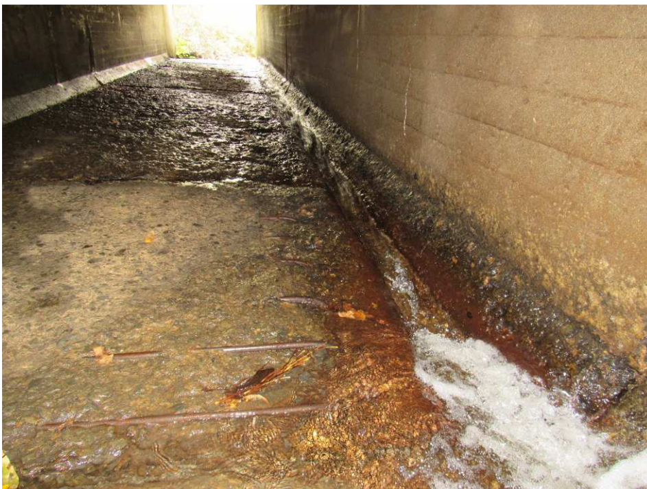
Photo 12 Key Feature: scour in floor of Rt 1 box culvert
