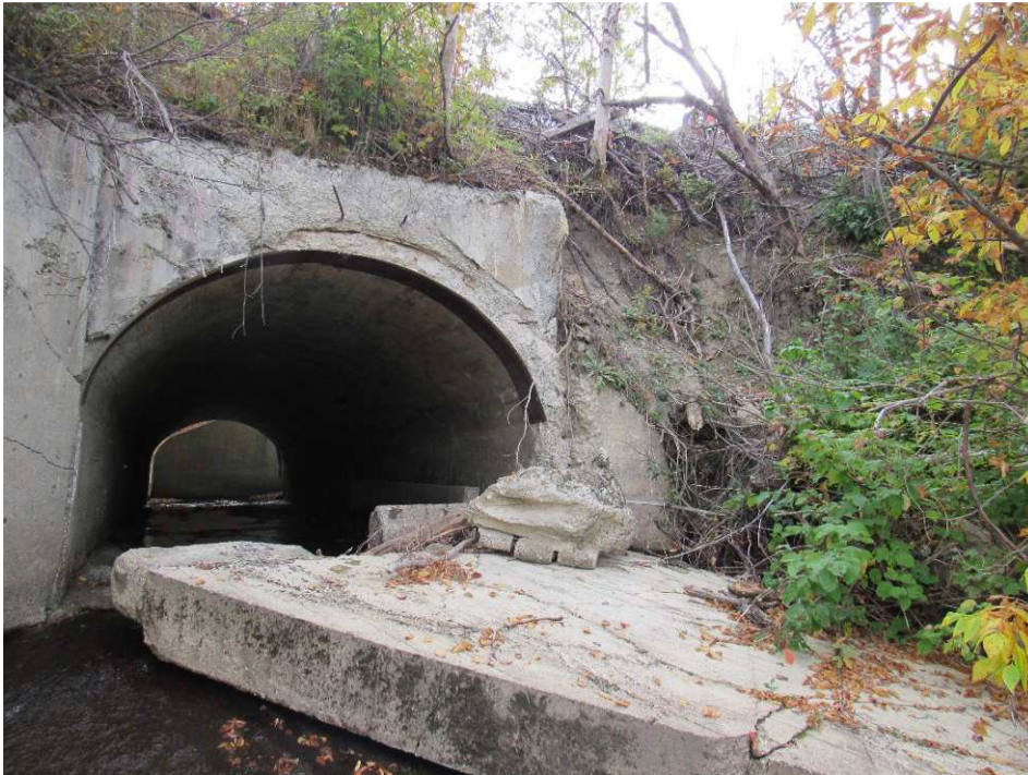
Photo 12 Key Feature: scour in floor of Rt 1 box culvert
