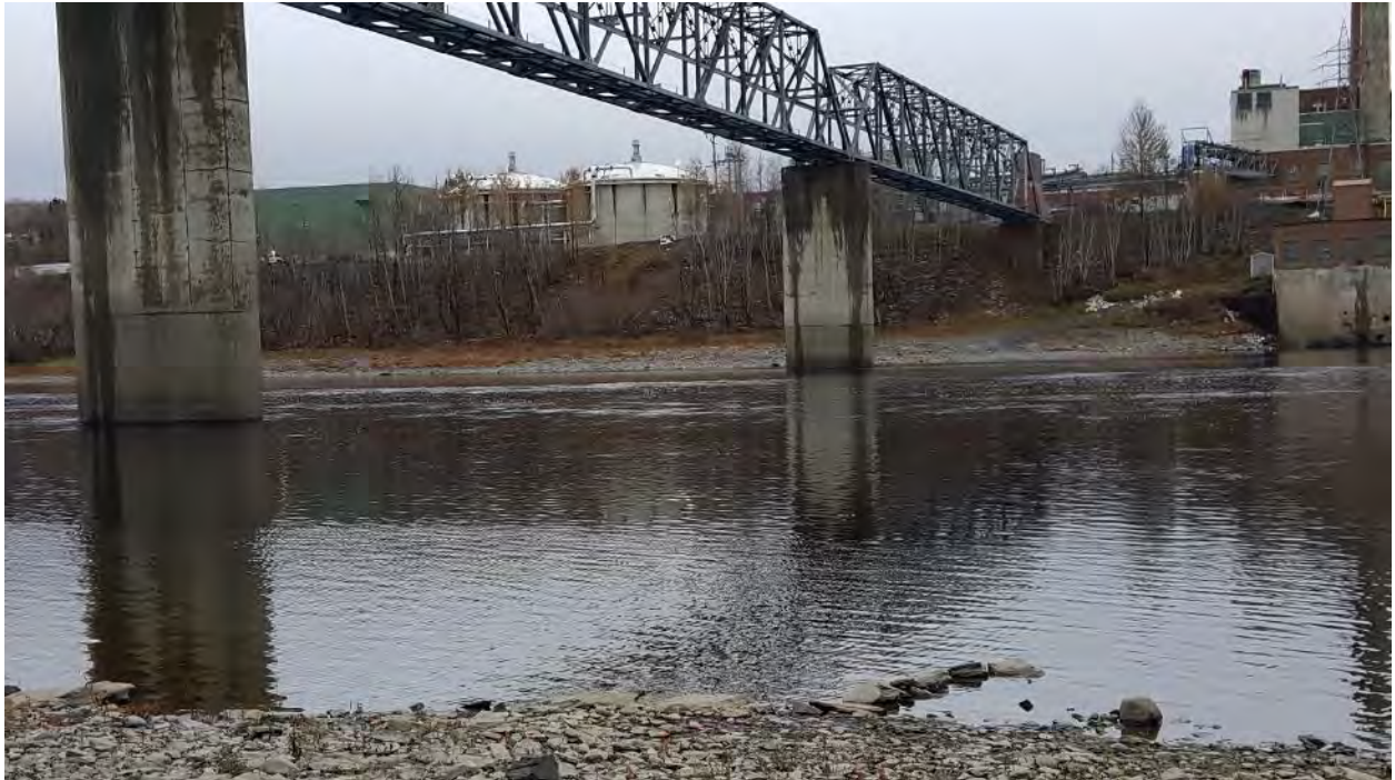
Figure 12. Twin Rivers Utility Bridge with rounded piers.
