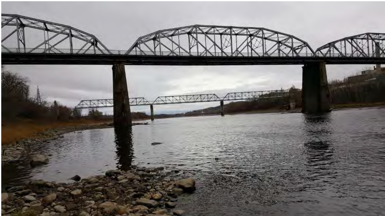
Figure 4. Looking downstream at International Bridge and Twin Rivers Utility Bridge
