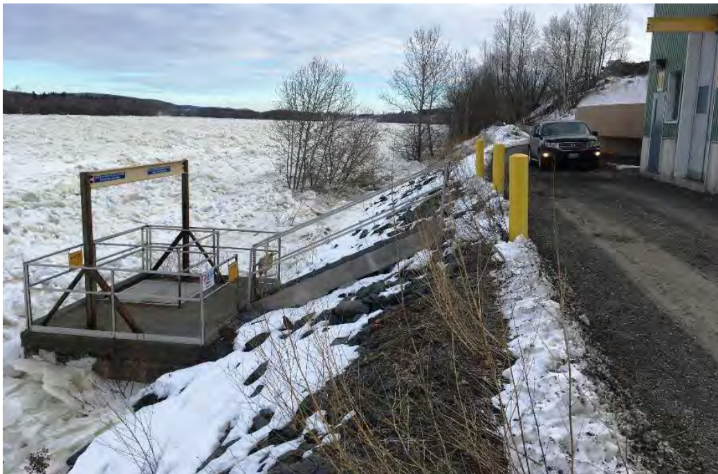
Figure 16. Water and ice at Twin Rivers manhole, spring, 2019
