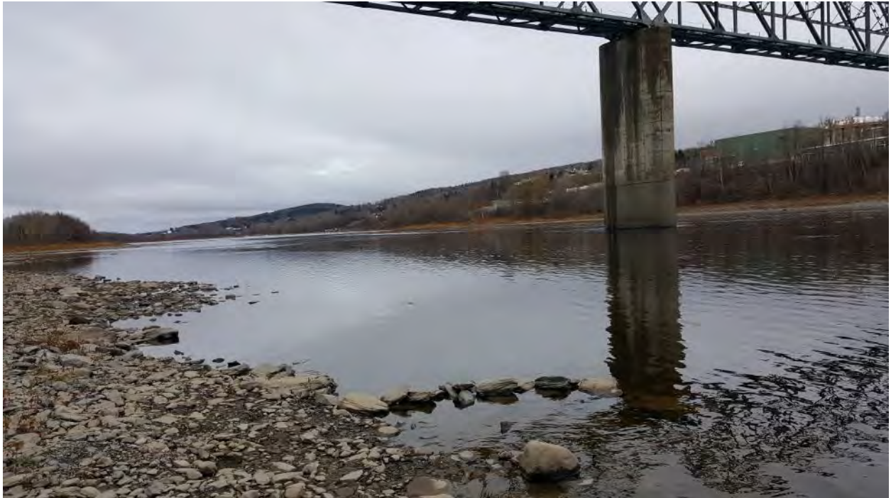
Figure 6. Twin Rivers Utility Bridge and downstream river reach
