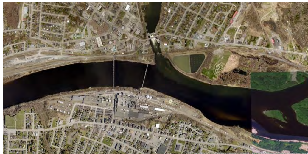
Figure 20. Aerial view of existing bridges and Madawaska River junction
