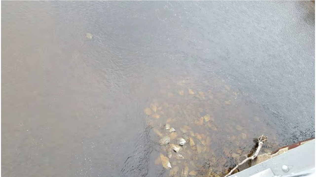
Figure 34. Riprap placed at nose of existing pier
