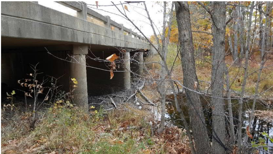
Figure 10. Upstream face of bridge from south side.
