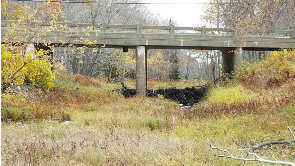
Figure 9. Boom Bridge from downstream
