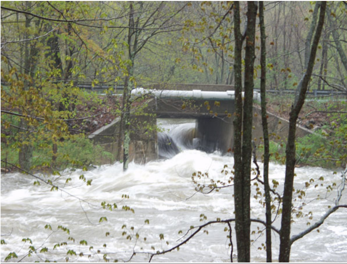
Figure 4 – Downstream side of bridge one day after “Mother’s Day Flood”
