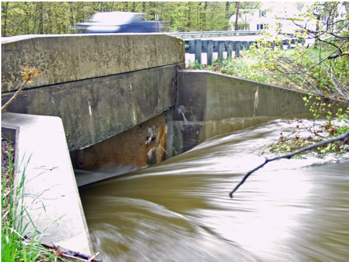
Photo 6 – Cape Neddick Bridge – Downstream Face of Bridge after FOR
