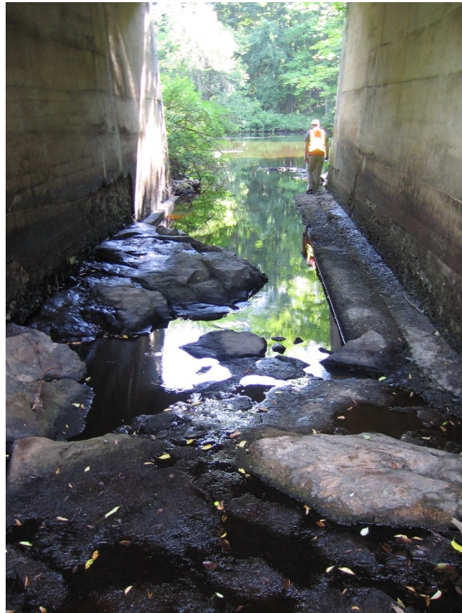
Photo 6 – Cape Neddick Bridge – Looking Downstream
