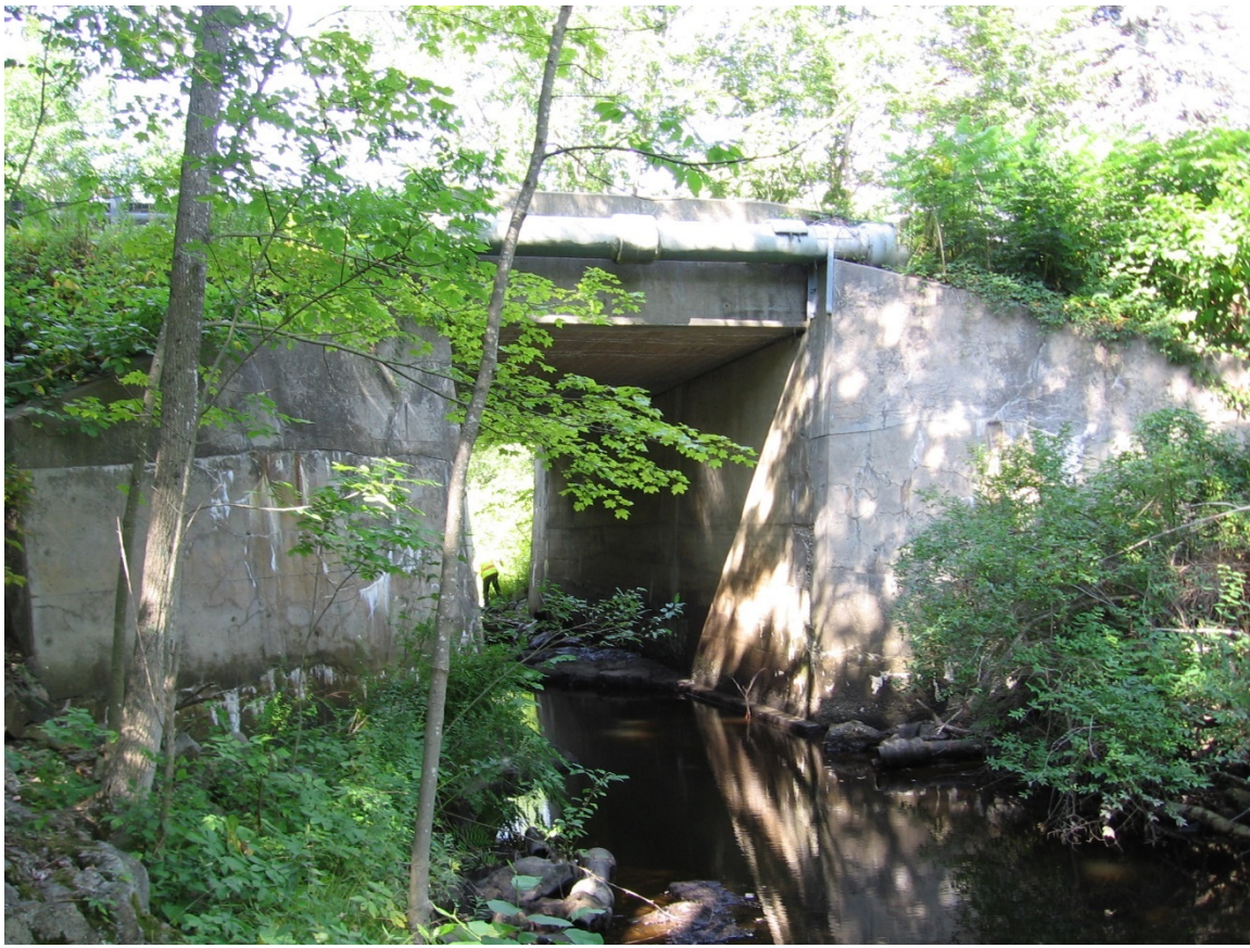
Figure 3 – Existing Structure Opening
