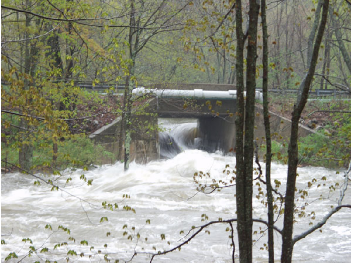
Photo 5 – Cape Neddick Bridge – Downstream Face of Bridge after FOR
