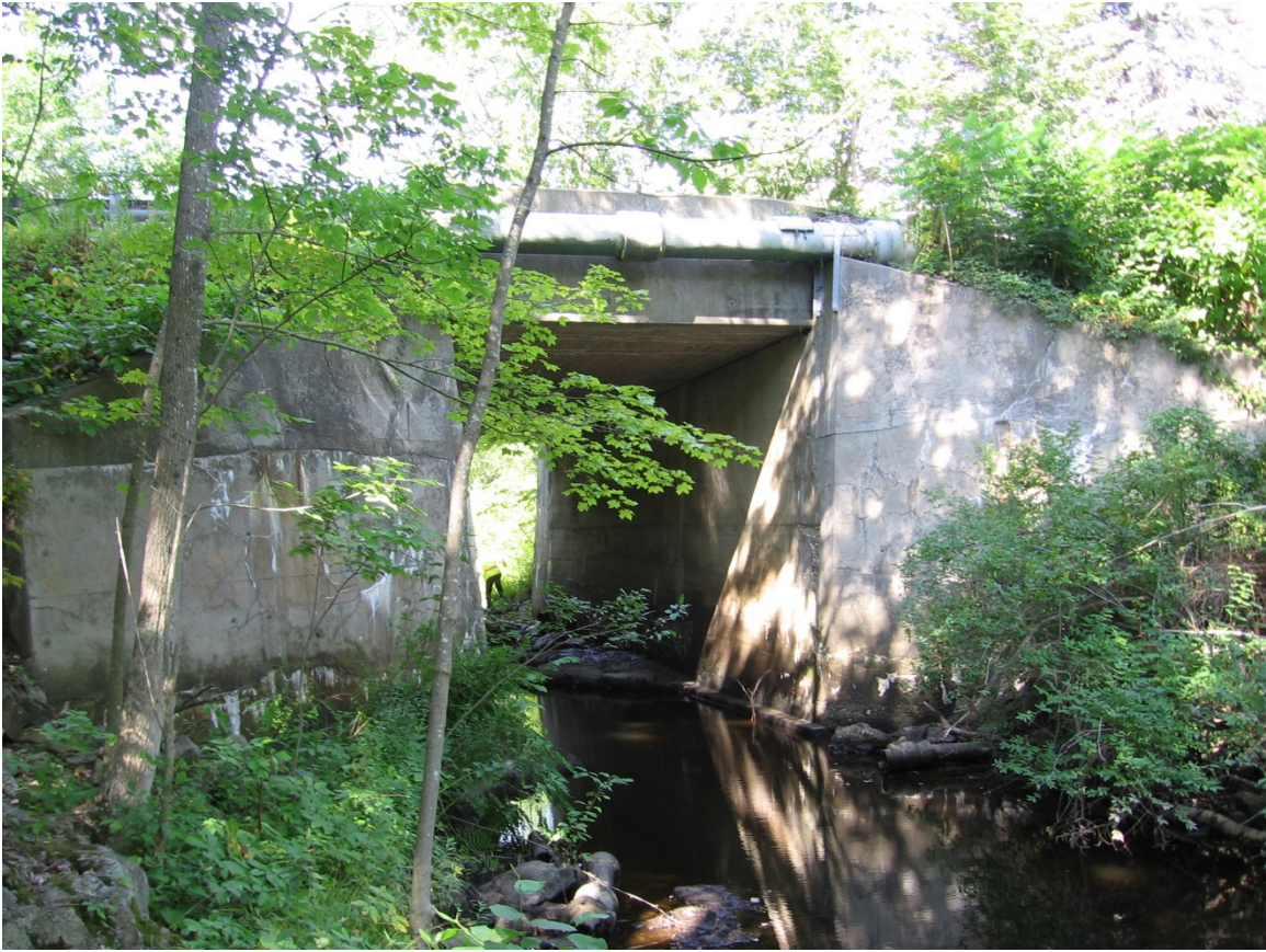
Photo 5 – Cape Neddick Bridge – Downstream Face of Bridge
