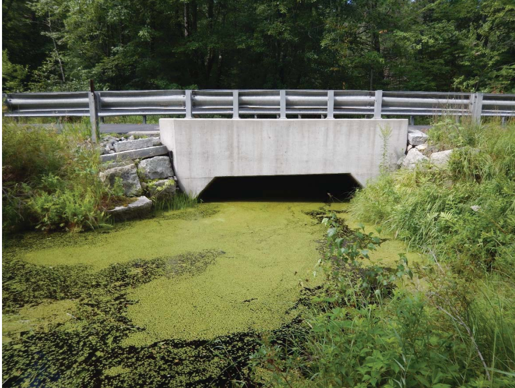
Photo 3: Upstream fascia (August 2018)
