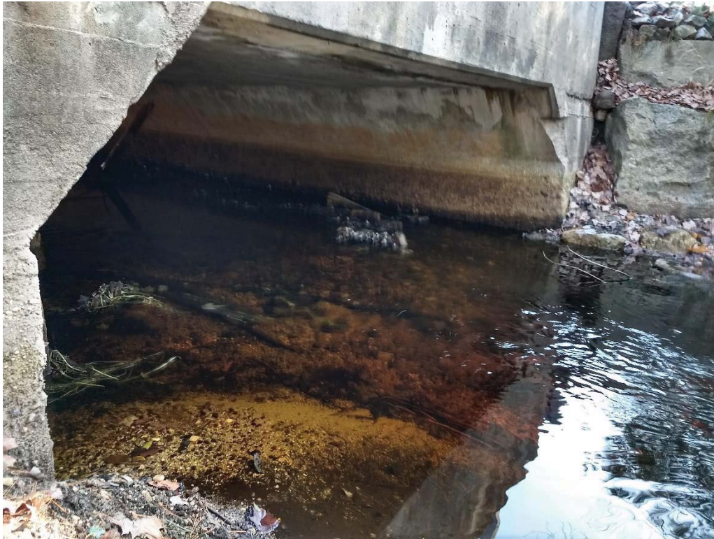
Photo 5: View at outlet (October 2018)
