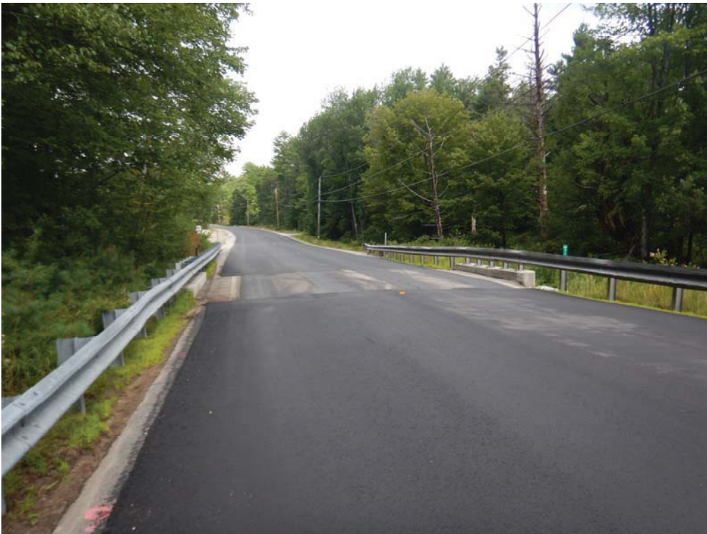
Photo 2: View from bridge, looking north
