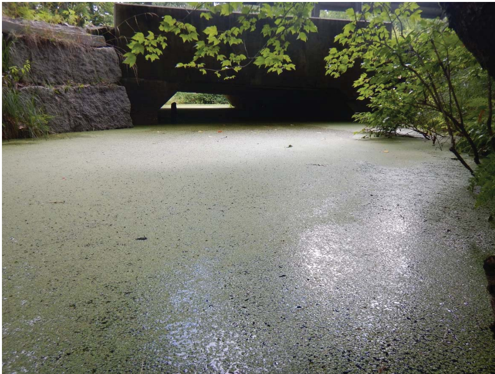
Photo 4: Downstream fascia (August 2018)
