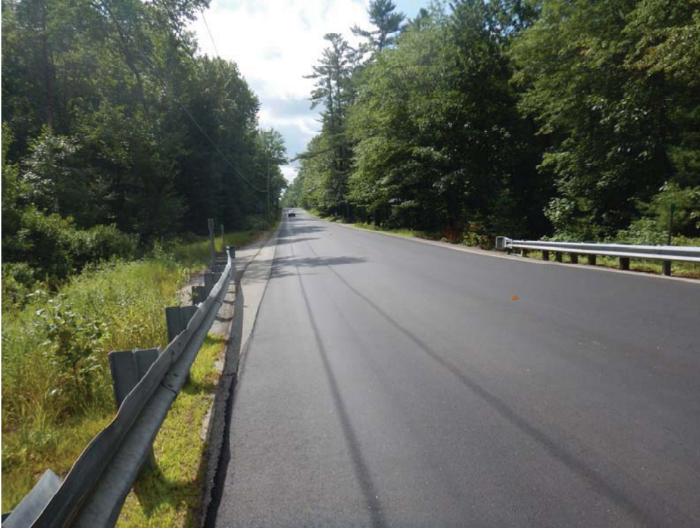
Photo 1: View from bridge, looking south
