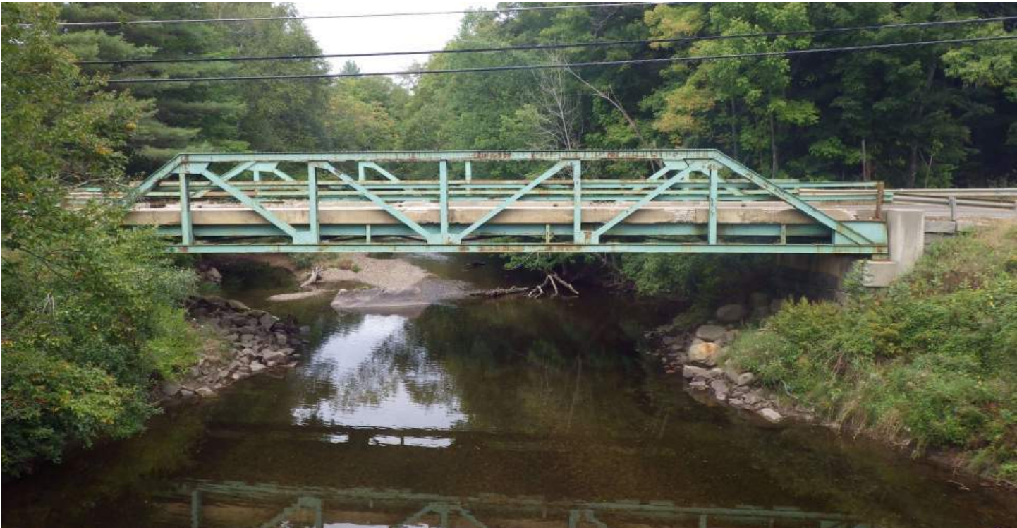
Photo 1 – Existing Structure– Looking Upstream
