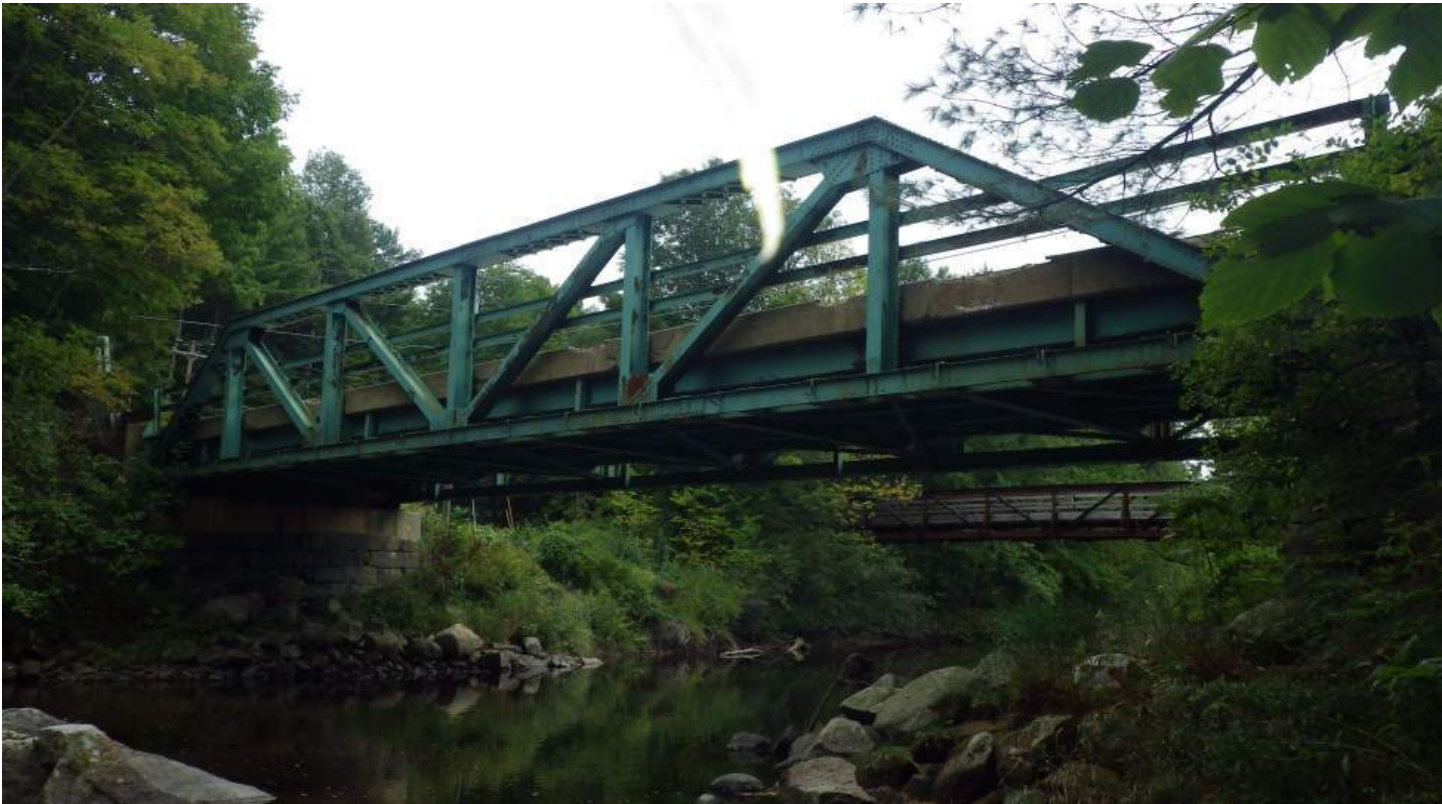
Photo 2 – Existing Structure and Snowmobile Bridge – Looking Downstream
