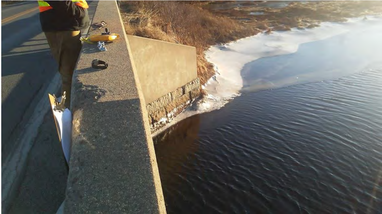
Figure 10. Water level measurements were taken from the lip of the rail, at the bottom edge of the angled portion at the center of each side of the bridge.
