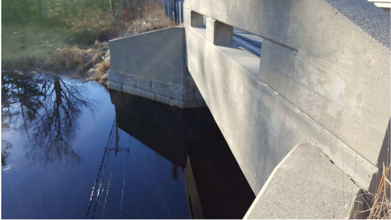
Figure 5. Downstream face of Marsh Bridge.
