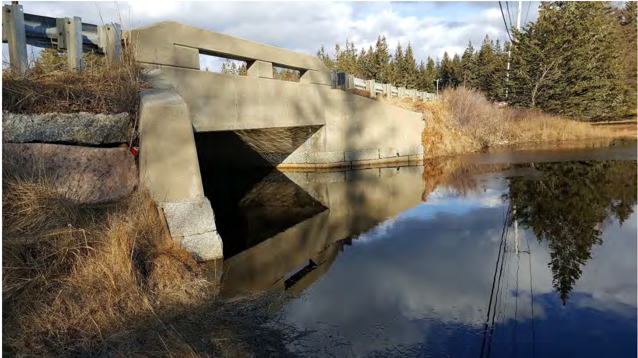
Figure 1. Marsh Bridge, upstream face.
