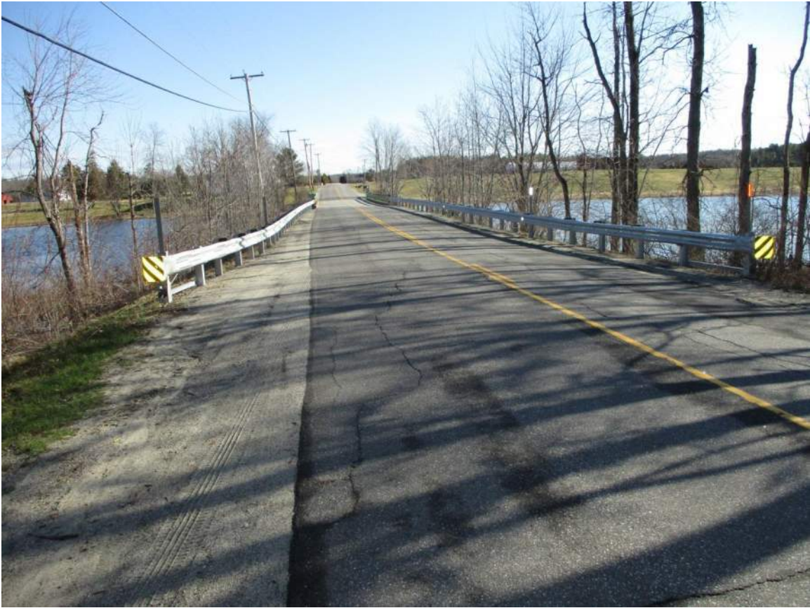
Photo 3 – Pond Road – South Approach
