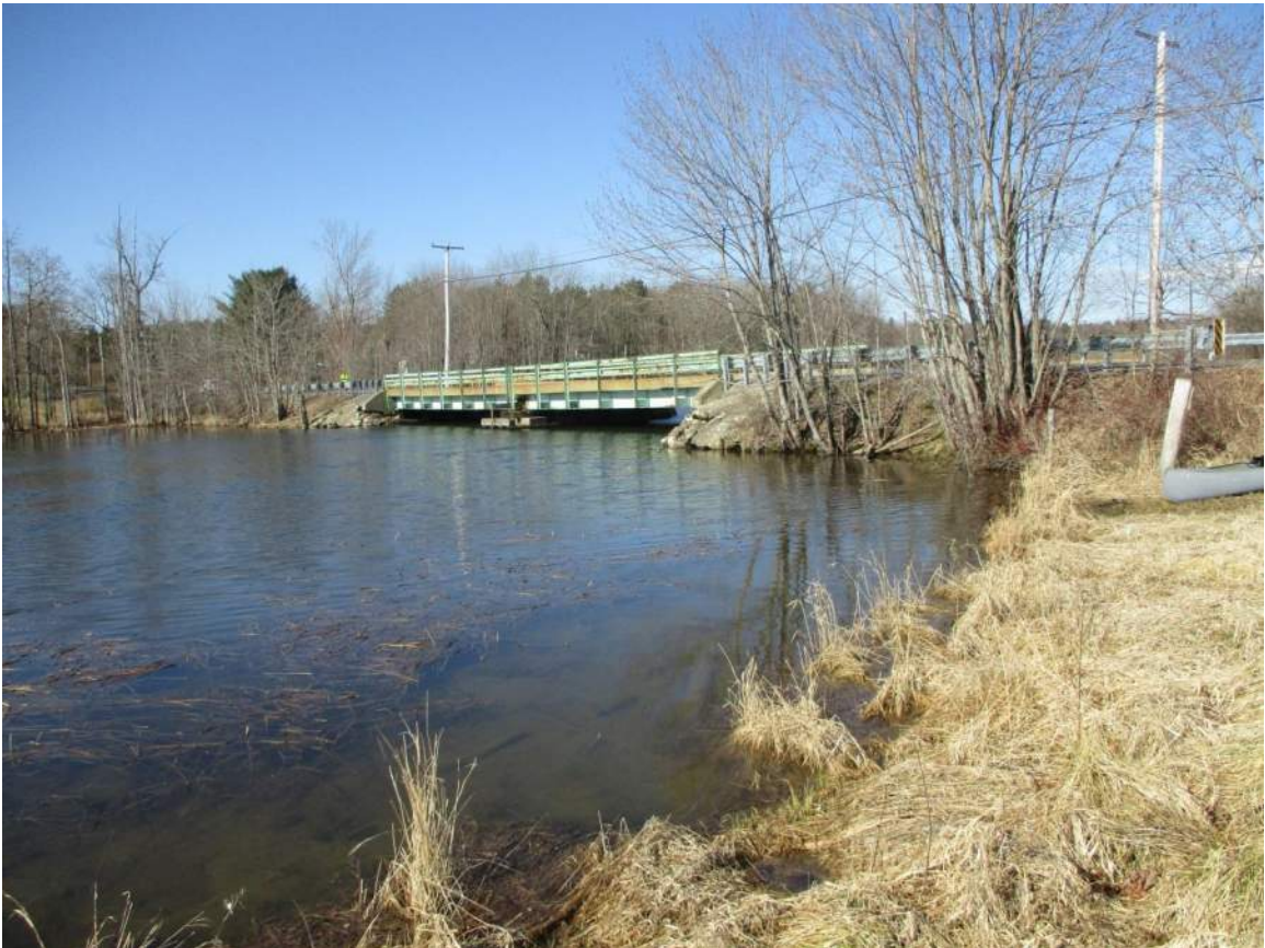
Photo 6 – Burnham Bridge – Downstream Face of Bridge
