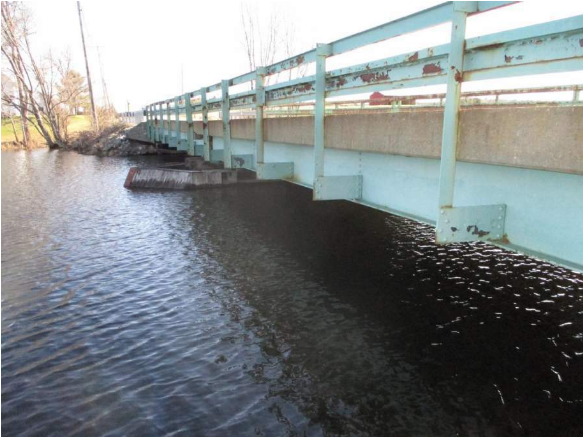
Photo 5 – Burnham Bridge – Upstream Face of Bridge
