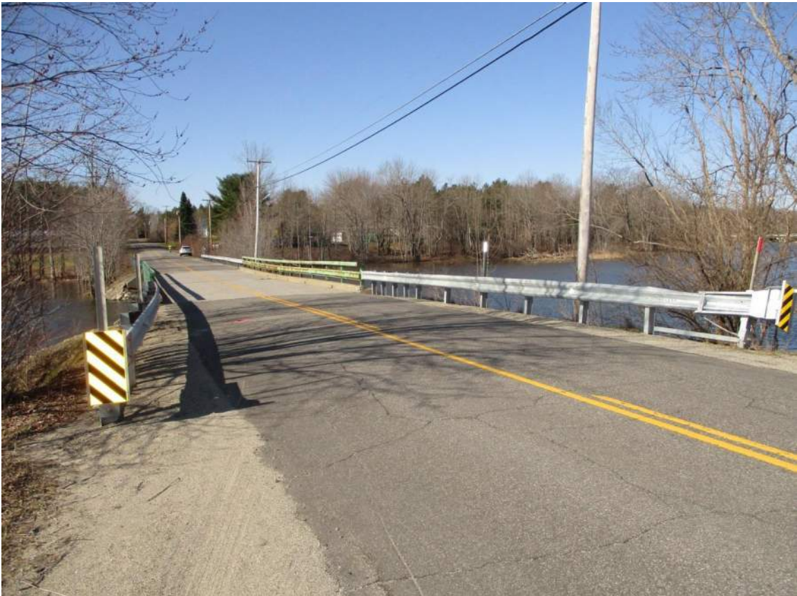
Photo 4 – Pond Road – North Approach
