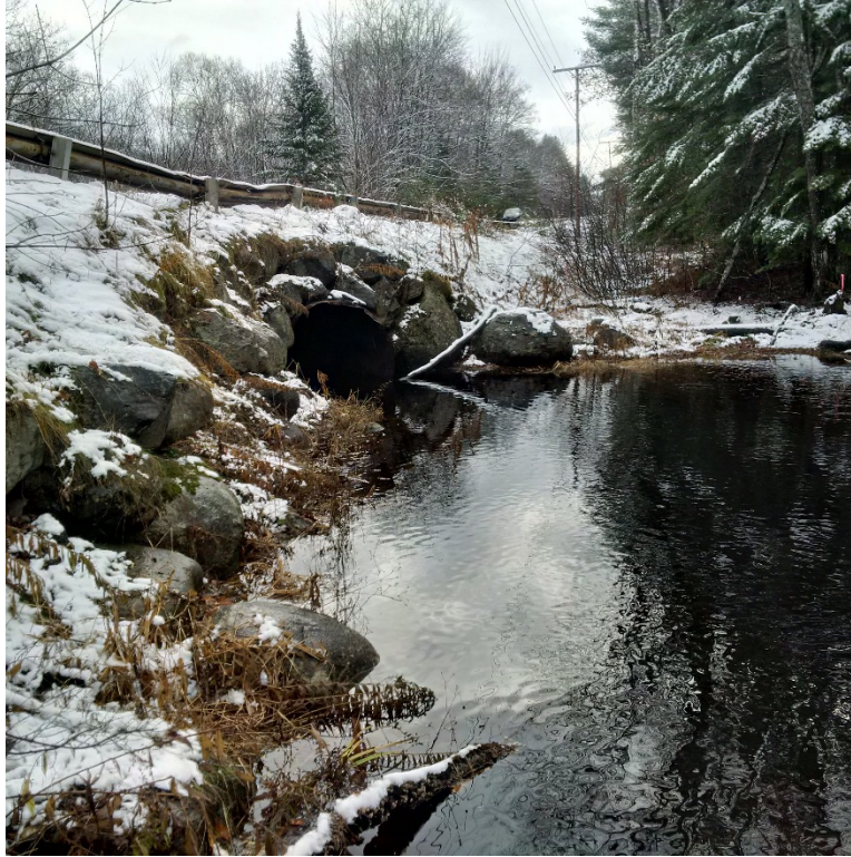
Photo 1. Culvert inlet (A. Walsh 11/23/2015).
