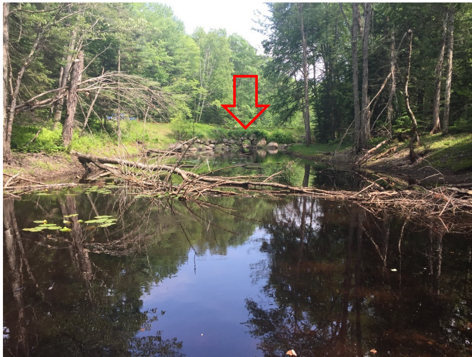
Photo 2. View looking downstream toward culvert inlet (red arrow) (8/7/2018).
