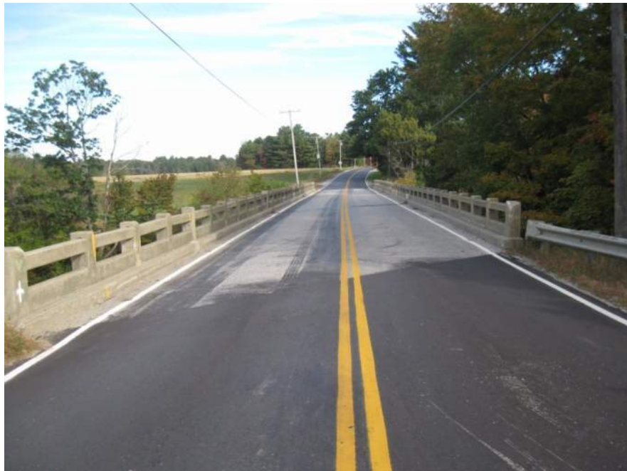
South Approach (Inspection Photo (10-5-2015))
