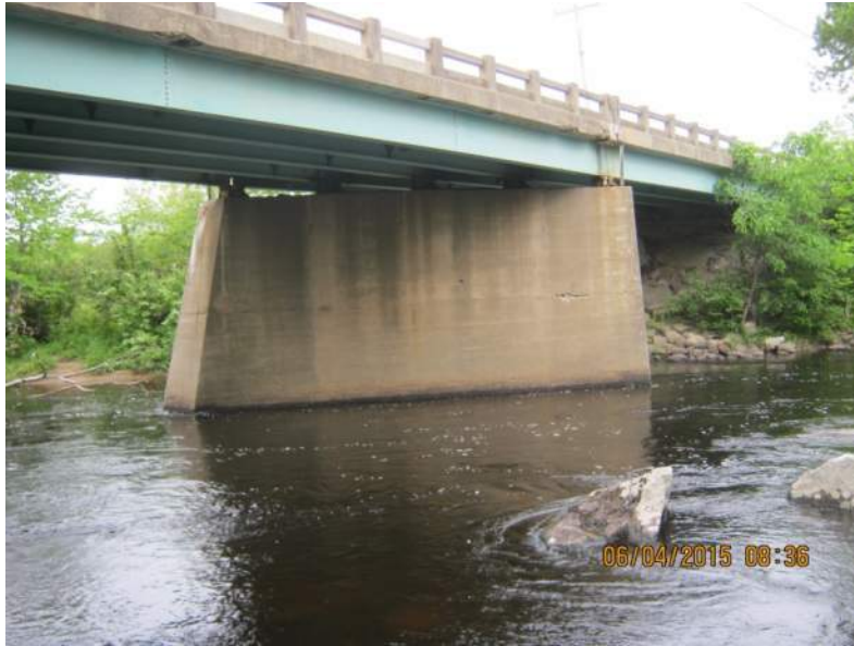
Downstream bridge view (Group Site Visit 6-4-15)
