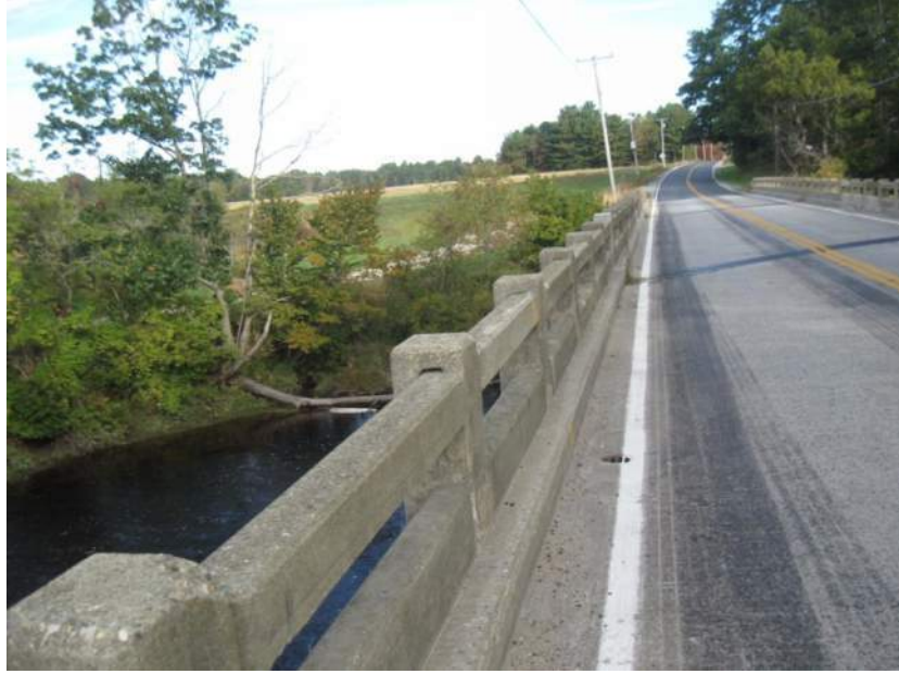
North Approach (Inspection Photo (10-5-2015))
