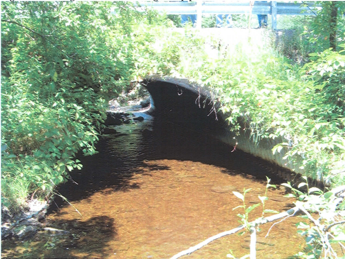
Figure 6: Looking upstream through pipe
