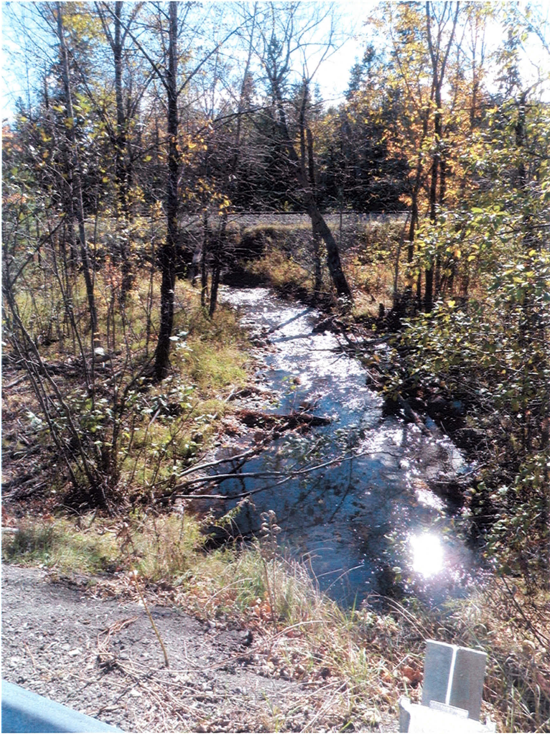
Figure 4: Railroad bridge downstream
