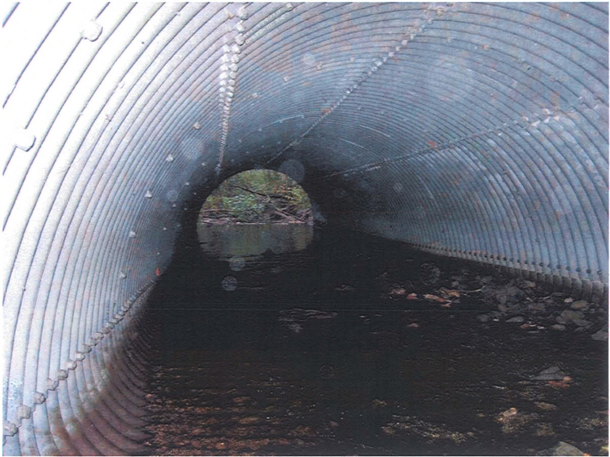
Figure 9: Good condition of top plates
