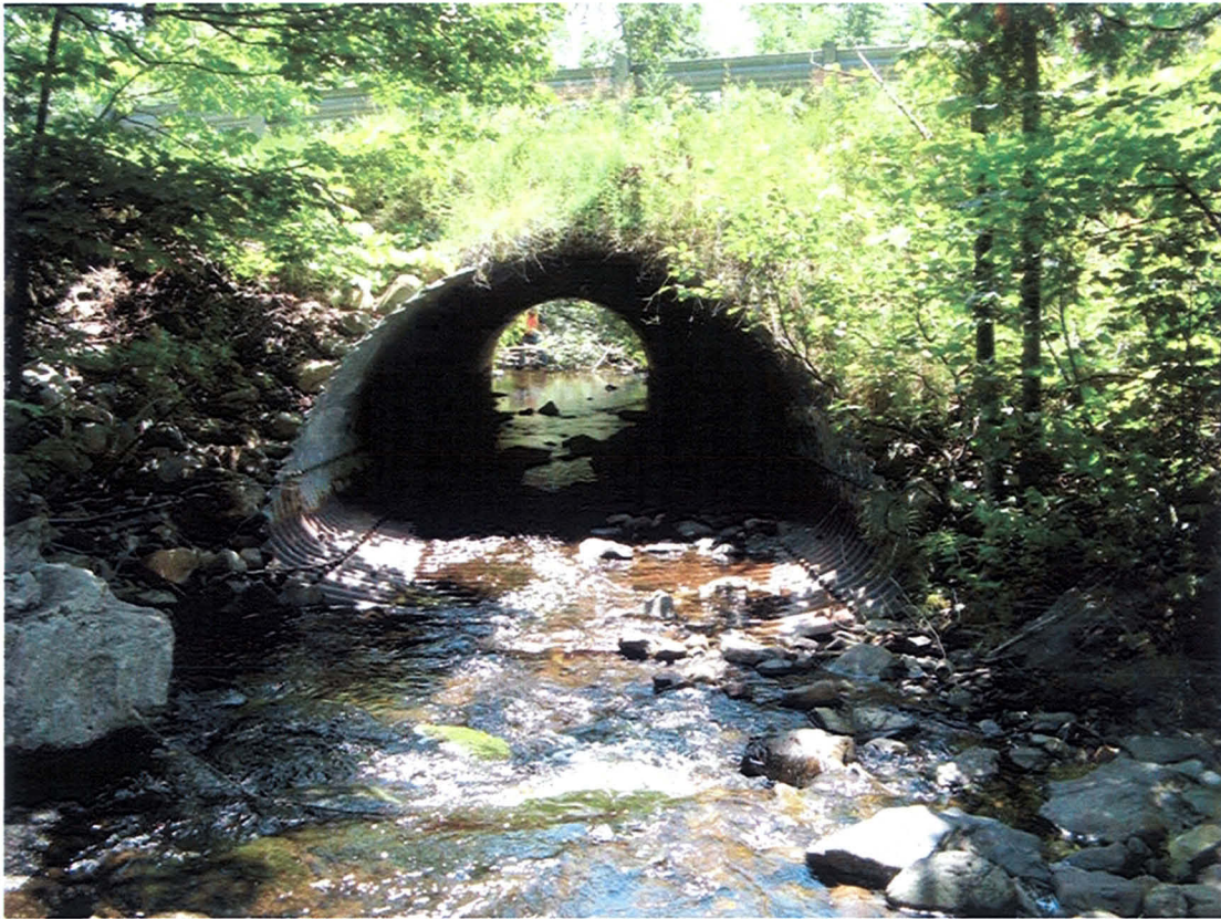
Figure 5: Looking downstream through the pipe
