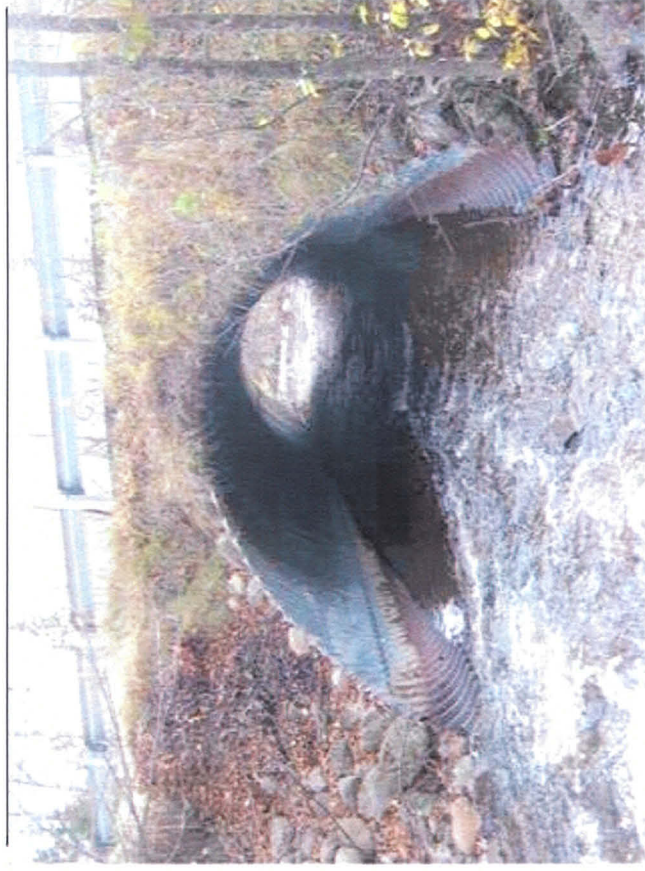
General view looking upstream - Note pipe bolt line indicates pipe is lifted at inlet
