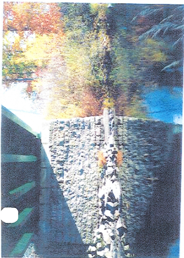
① looking at right abutment, note concrete cap, U.S.
