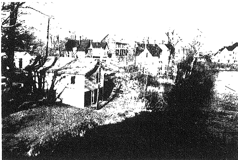
FIGURE 3 - Downstream of Portland Terminal railroad bridge - Westbrook. Note building in foreground - waters would approach top of basement window.
