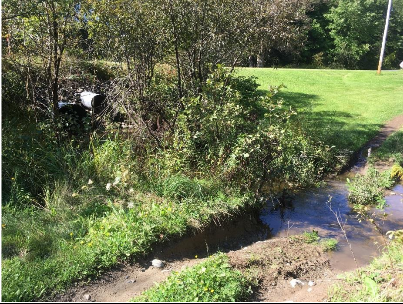
Figure 8E: Downstream ATV Crossing Showing Outlet
