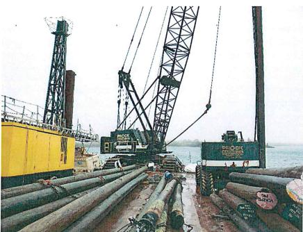
Photo 5: Link-Belt LS-518 crawler crane used to advance HP12x53 steel H-pile probe.
